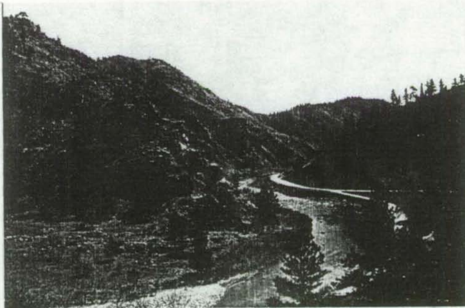
FIGURE 5.9 DOWNSTREAM VIEW SOUTHEAST TOWARD POUDBRE DAM SITE.
