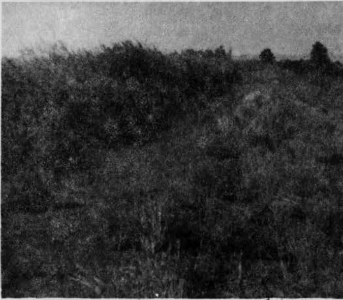
PHOTO 7.5-4 — THE CREST OF A DAM PARTIALLY OVERGROWN AND OBSCURED DUE TO EXCESSIVE BRUSH GROWTH
