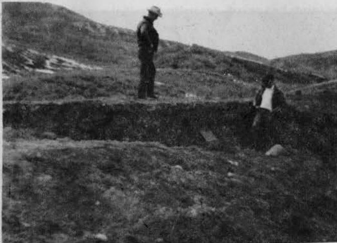
PHOTO 7.5-1.a — VERTICAL DISPLACEMENT ON CREST.
