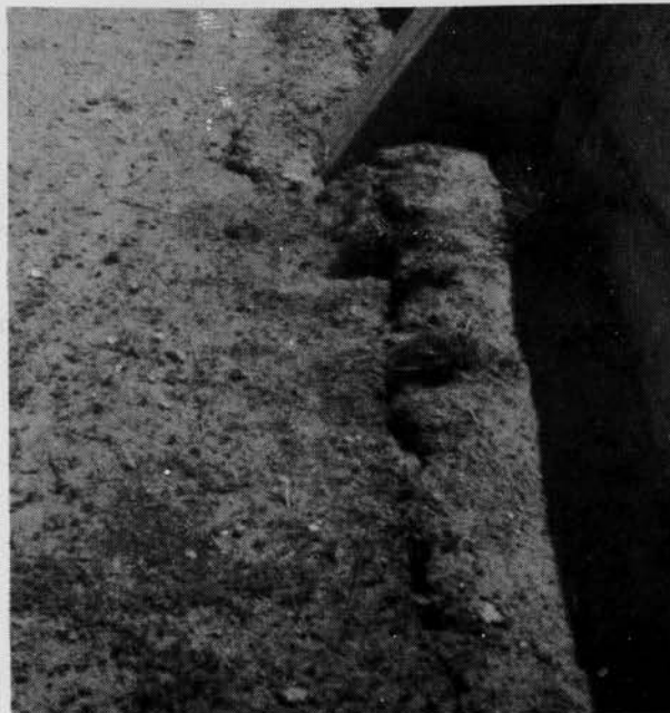
PHOTO 8.5-3 — LONGITUDINAL CRACKING
