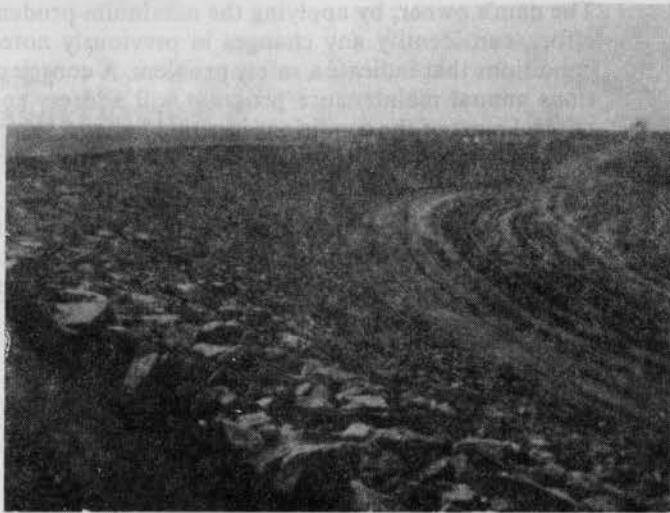
PHOTO 6.1 — EXCELLENT UPSTREAM FACE. Note uniform surface of riprap protection.
