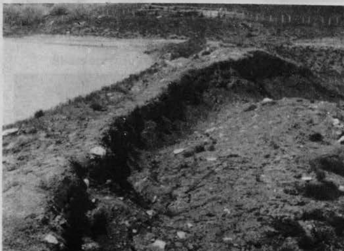
PHOTO 7.5-1.b — VERTICAL DISPLACEMENT ON THE CREST OF A DAM. This vertical movement was associated with a slip on the downstream face.
