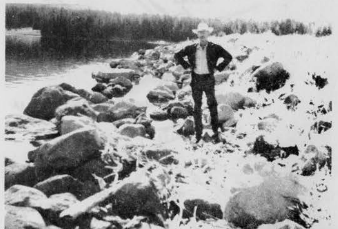
PHOTO 6.5-6 — SLIDE AT UPSTREAM SLOPE. Note water line alignment.
