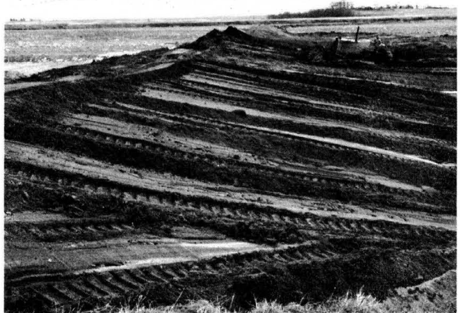
Figure 5. Construction of dam D-2, site No. 1.
