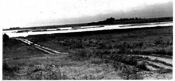
5 5 Figure 10. Flood flow destroying structures at site No. 1 on July 24, 1965. do
