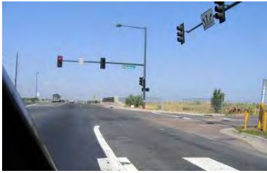
56 th Avenue at Havana Street, a bridge over Havana Interceptor in the distance. Looking northwest
