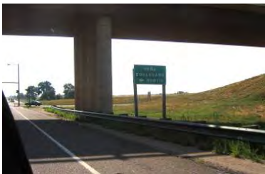
Under Peña Boulevard Bridge Looking southeast
