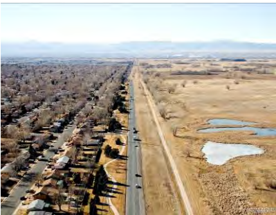
56 th Avenue, looking west
