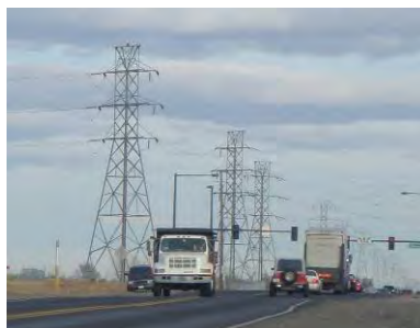
Xcel transmission towers in the corridor
