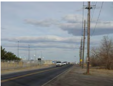
Xcel electric lines in the corridor
