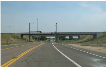
56 th Avenue and Peña Boulevard Interchange—looking east
