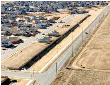
Parkfield neighborhood on the upper left. Looking southwest over 56 th Avenue
