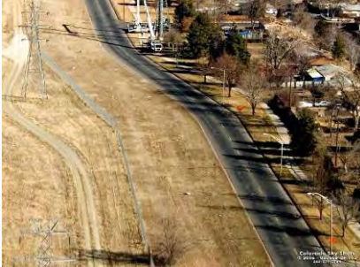
Two-lane section of 56 th Avenue from Peoria Street to Peña Boulevard—looking east
