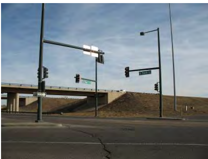
56 th Avenue at Peña Boulevard Southbound Ramp—looking southeast
