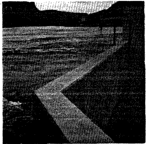
Photo 20. Retaining Wall Constructed during 1983 to Protect Ute Water Conservancy District Pump Station located on Colorado River Near Grand Junction (Note: 1984 Floodwater Nearly Overtopped Wall).
