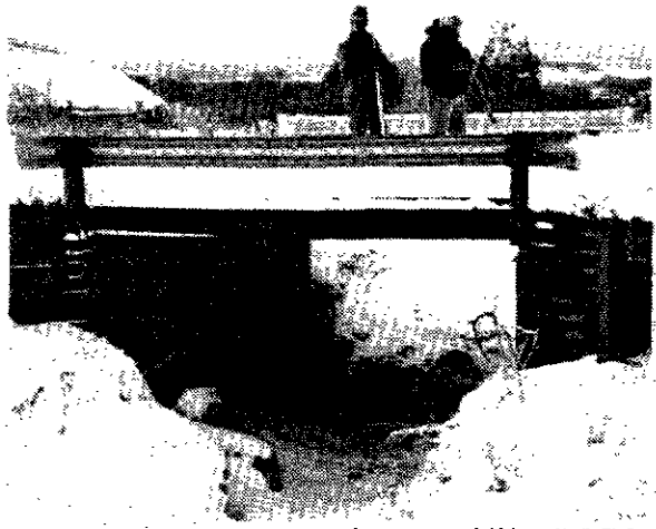
Photo 12. Beaton Creek Bridge in Montrose County.
