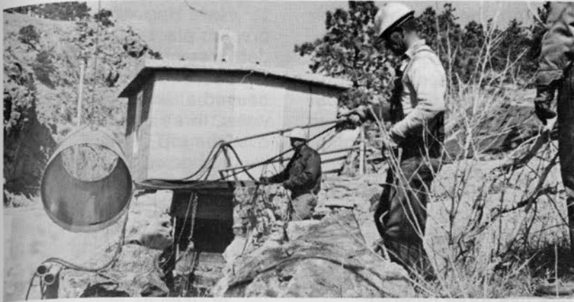
Installing new inlet pipe to the plant in 1959 (left and below)
