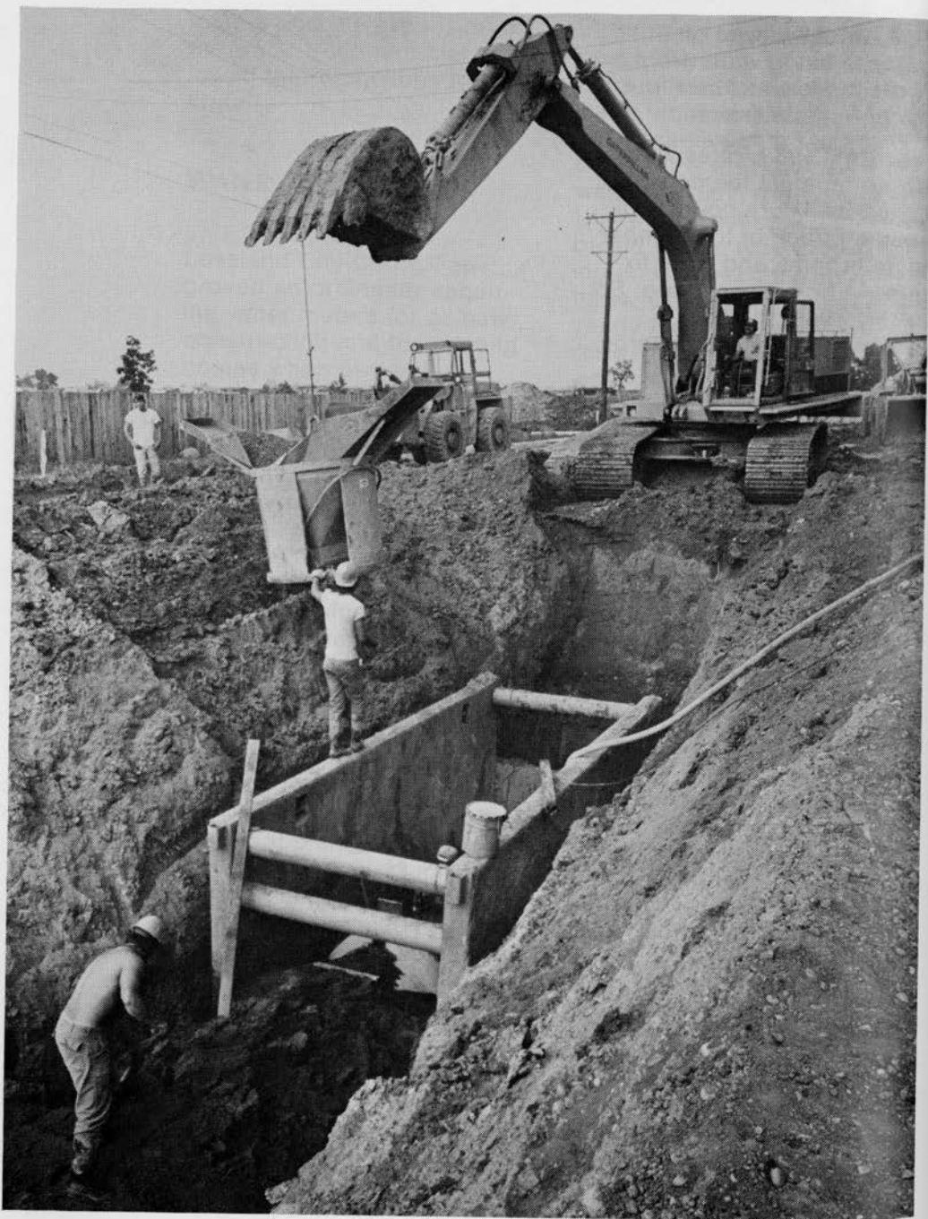
Installing a manhole on North Madison Avenue - 1982
