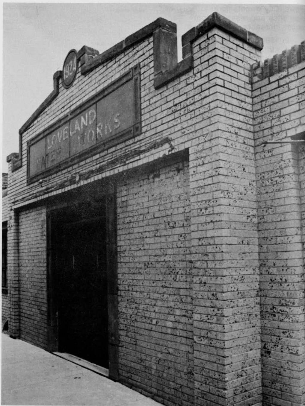
Rapid Sand Filter Building - built in 1924
