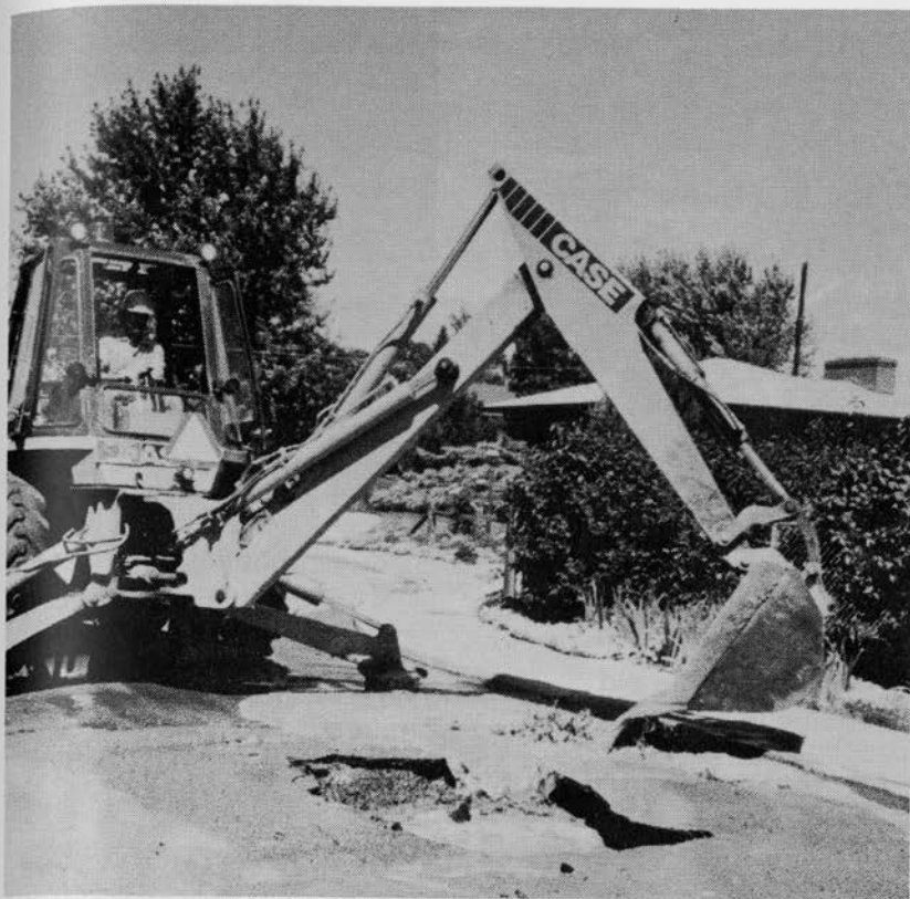
Ray Frank repairing a leak on Connecticut Avenue
