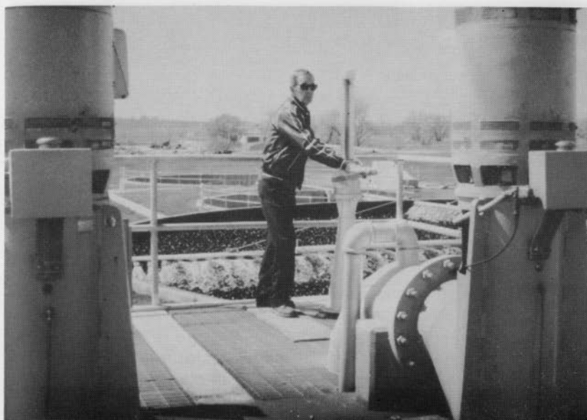
Retired Operator Jerry Ulin at the controls of the trickling filter
