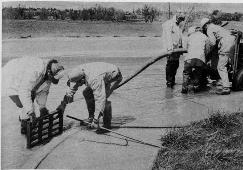
Cleaning out a clogged storm drain
