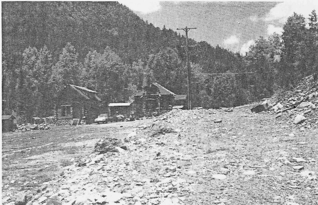
Figure 5. Looking north toward the most seriously affected properties. The main haulage adit is in the trees on the right of the picture.
