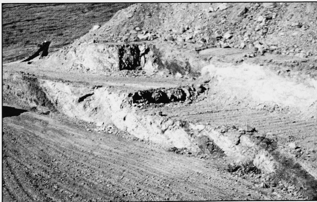
Figure 14. Middle part of Morrison Formation exposed in a basement excavation in northwestern Douglas County. The bedrock consists of steeply dipping layers of dark-red claystone, light-gray claystone, and medium-brown sandstone. The claystone beds tend to be moderate- to high-swelling, while the sandstone beds are typically non-swelling.
