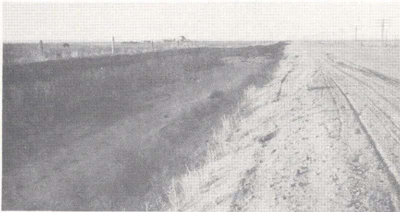
Looking north in wash along west side of Highway 85 about 2-1/2 miles north of Pierce. Length of wash 1500 feet, depth about 9 feet.
