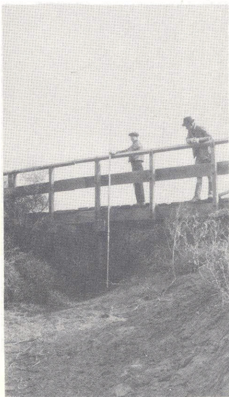
Bridge over Laramie-Poudre Ditch about 1-3/4 miles east of Nunn. Important critical section owing to small area and weeds.
