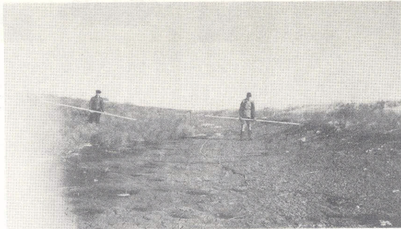
Looking east down Laramie-Poudre Ditch about 1/4 mile east of Nunn. Shows weeds in ditch bottom. Bottom width 20 feet.
