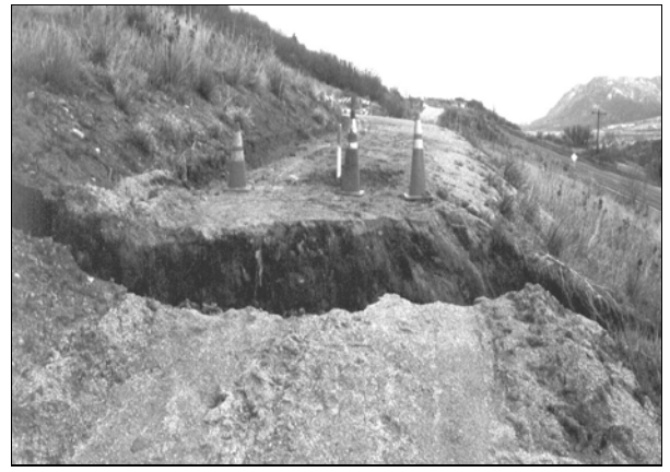
Landslide toe damages roadway (left) while the scarp damages bike path (right) in Colorado Springs. Photos by John Himmelreich.
