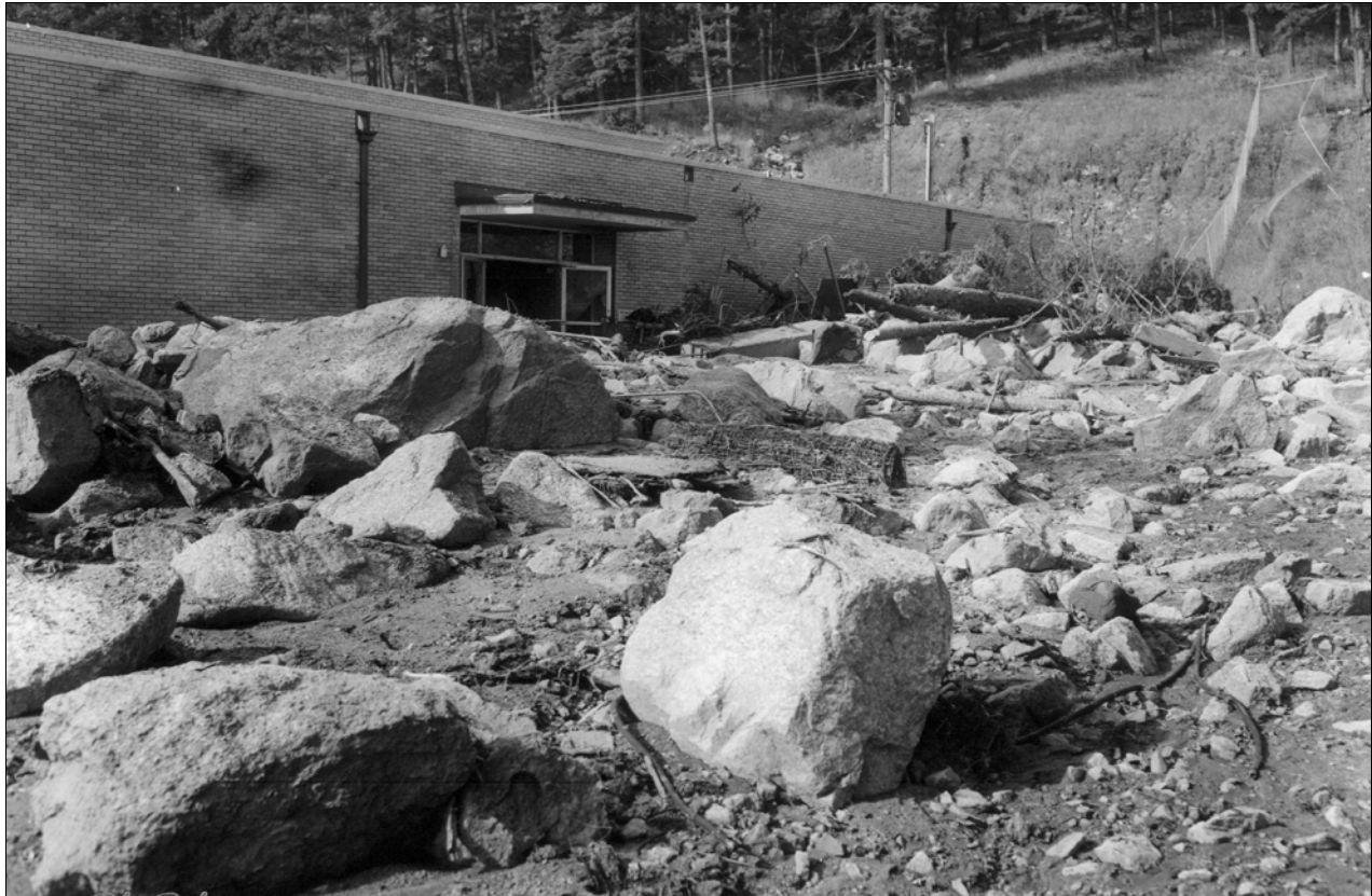
Debris flows from fatal July 24, 1965 storm damage the Hippo House at Cheyenne Mountain Zoo. Photo courtesy of the Pikes Peak Library District.
