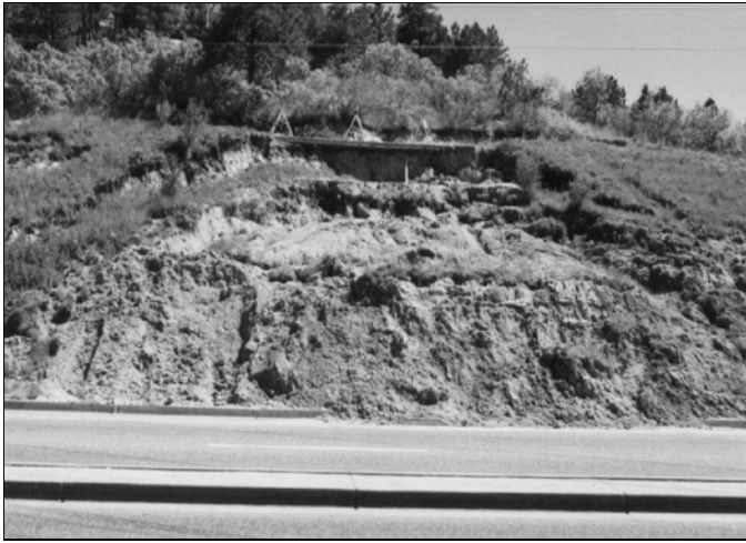
Slump encroaches on roadway and jeopardizes bike path (left). Photo by John Himmelreich. Landslide closes two lanes on Interstate 25 (right). Photo courtesy of the Pikes Peak Library District.
