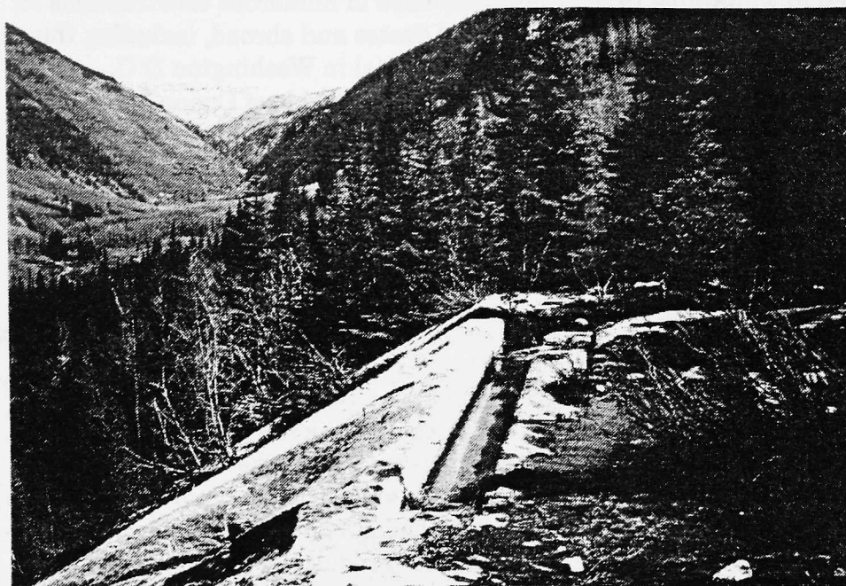
Figure 2: A view, looking down-valley to the north, from the upper bench of the Colorado - Highland quarry which operated on site in 1912. Not visible in this photo is a four foot cutwall at back of quarry cut and old cable used to lower blocks to loading area below. Bench also extends to south of photo vantage-point.
