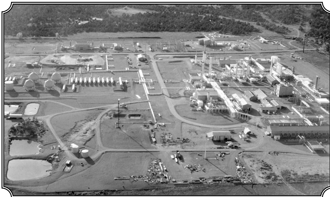
WILLIAMS GAS PROCESSING PLANT, IGNACIO, COLORADO
