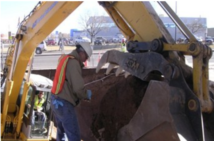
Grab soil sampling from beneath the tanks.
