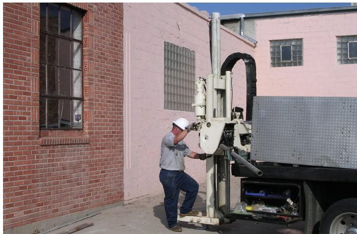
Direct-push soil sampling in the area of a former tank basin.
