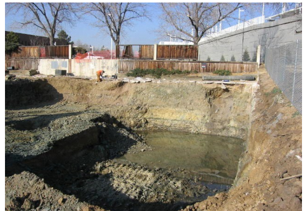
Petroleum-Impacted Soil Excavated
