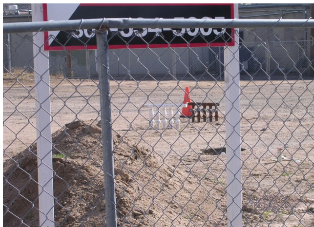
Remediation System Installed
