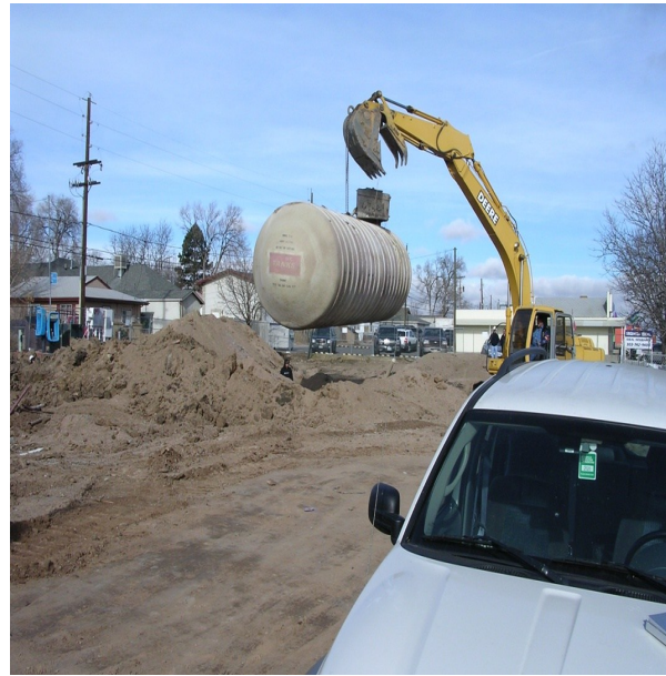
Storage Tank Removal
