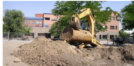
Tank removal is a separate program within the Redevelopment Fund
