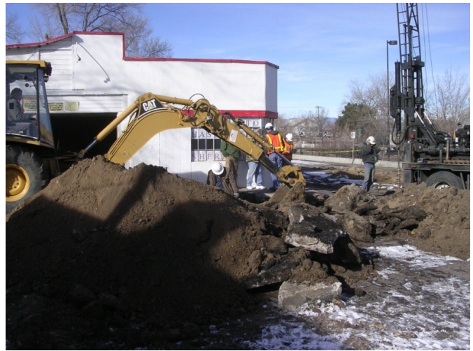
Storage Tank Removal/Impacted Soil Excavation
