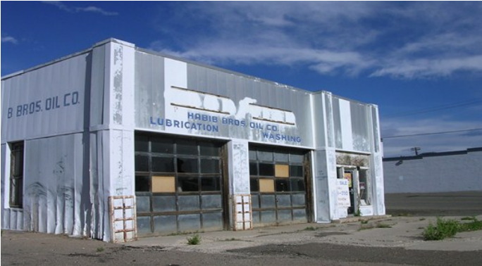
Blighted property in need of redevelopment.
