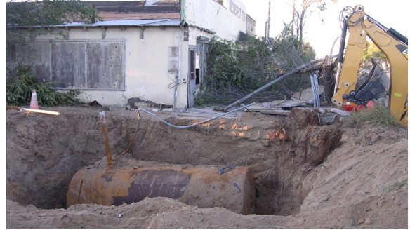
Underground storage tank removal and the start of redevelopment.
