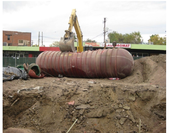
Underground Storage Tank Removal
