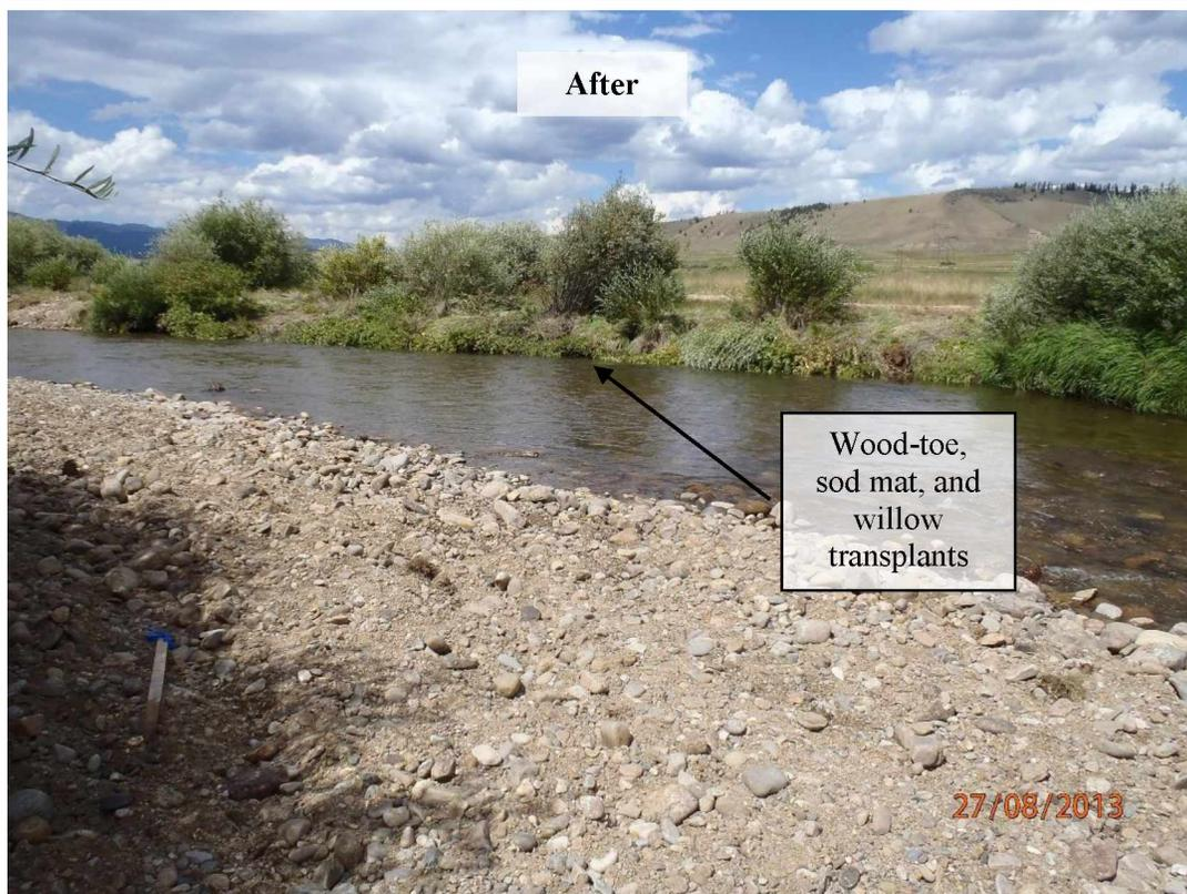
**Figure 1.3.** Before vs. after photos showing the treatment of excessive bank erosion with wood-toe, sod mats, and willow transplants on the Upper Arkansas River.
