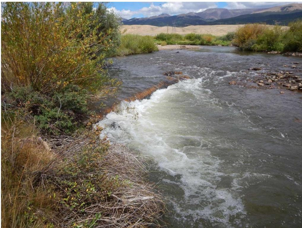
**Figure 7.4.** Typical log-vane structure used during habitat restoration on the Upper Arkansas River.
