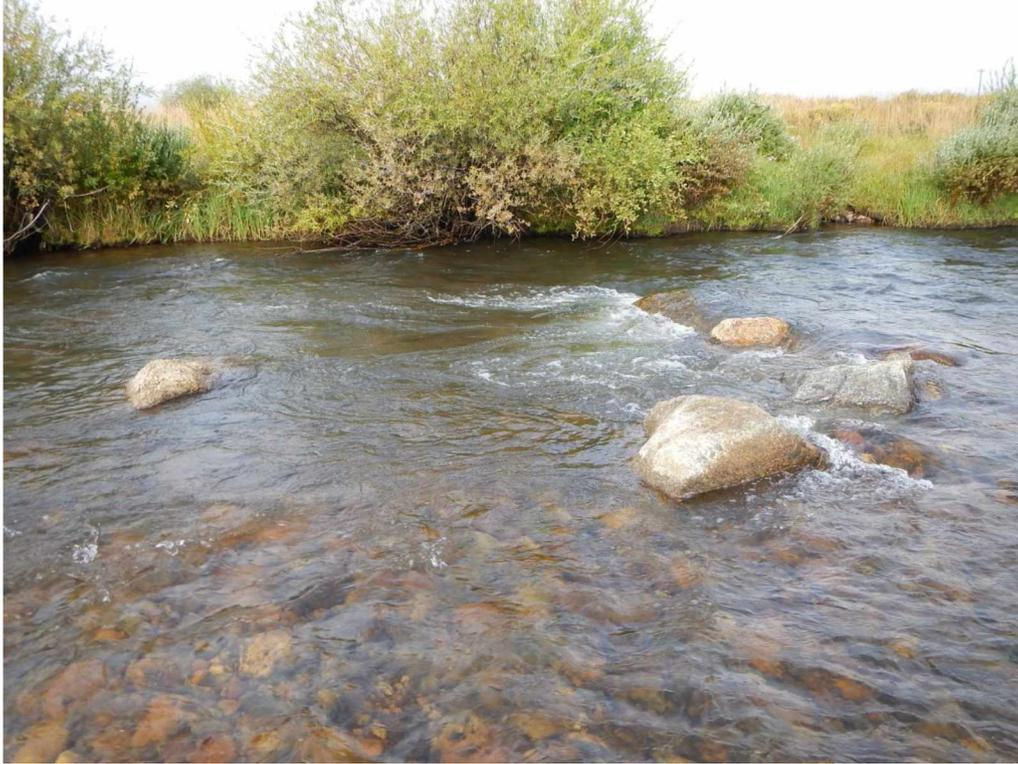
**Figure 7.1.** Typical boulder cluster structure used during habitat restoration on the Upper Arkansas River.
