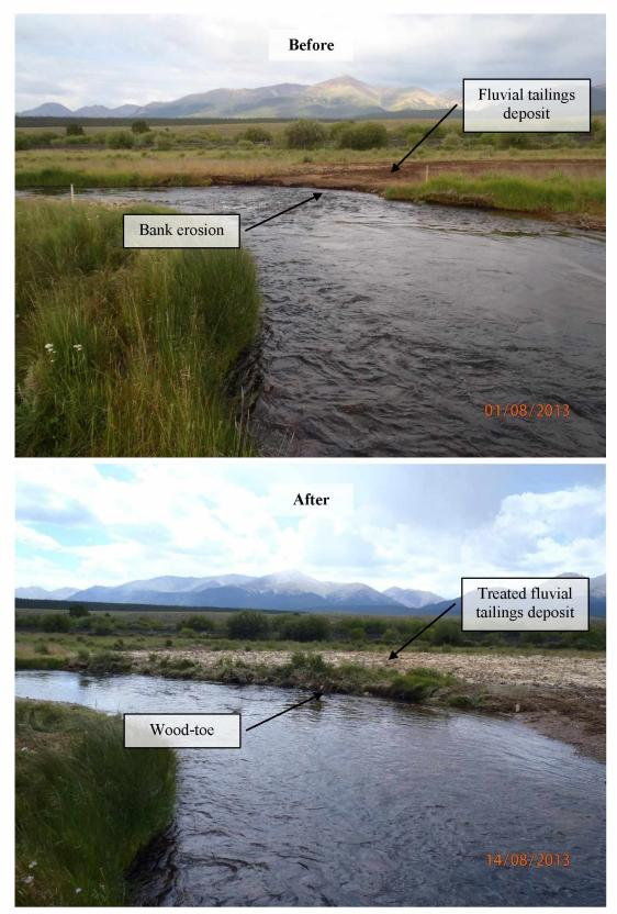
Figure 1.6. Before vs. after photos showing treatment of a fluvial tailing deposit and stabilization of an eroding bank with wood-toe on the Upper Arkansas River.
