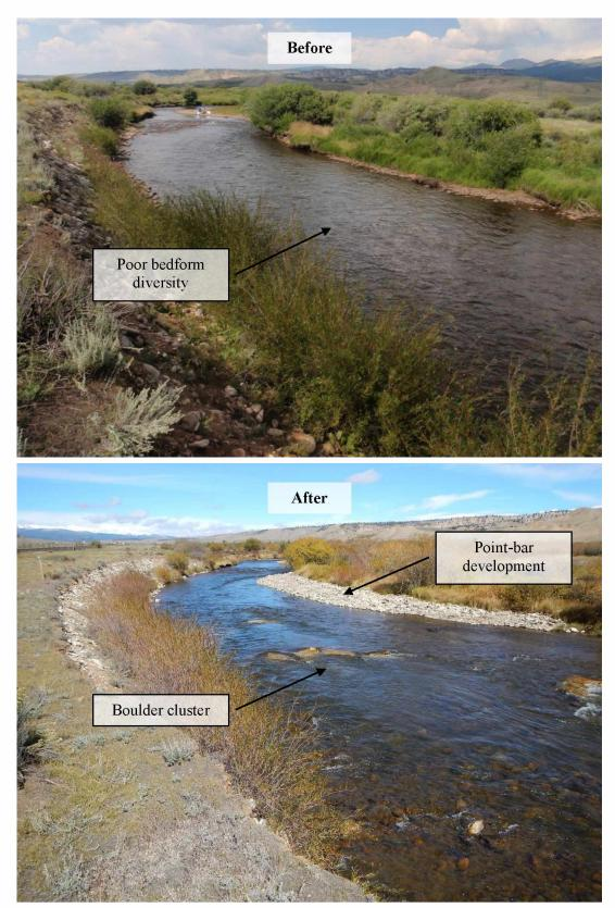
Figure 1.5. Before vs. after photos showing treatment of a reach characterized by poor bedform diversity with point-bar development, pool development, and boulder clusters on the Upper Arkansas River.
