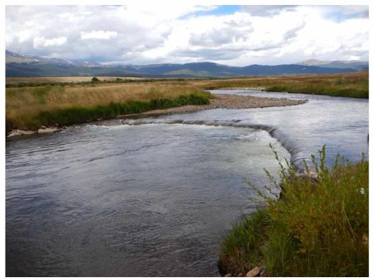
Figure 7.5. Typical log/rock-vane structure used during habitat restoration on the Upper Arkansas River.
