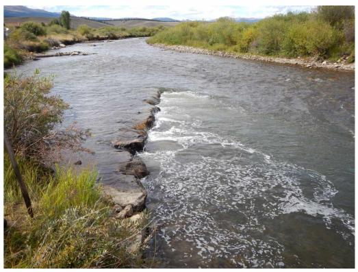
Figure 7.3. Typical rock-vane structure used during habitat restoration on the Upper Arkansas River.
