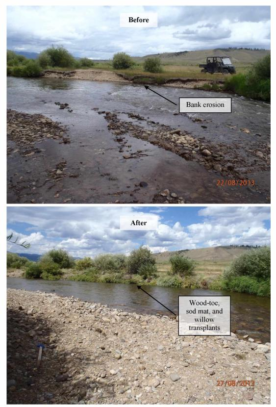
Figure 1.3. Before vs. after photos showing the treatment of excessive bank erosion with wood-toe, sod mats, and willow transplants on the Upper Arkansas River.
