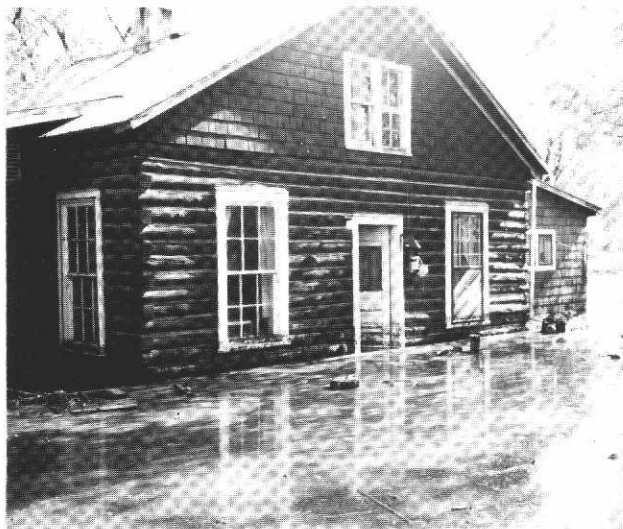
Flood Damaged Property
