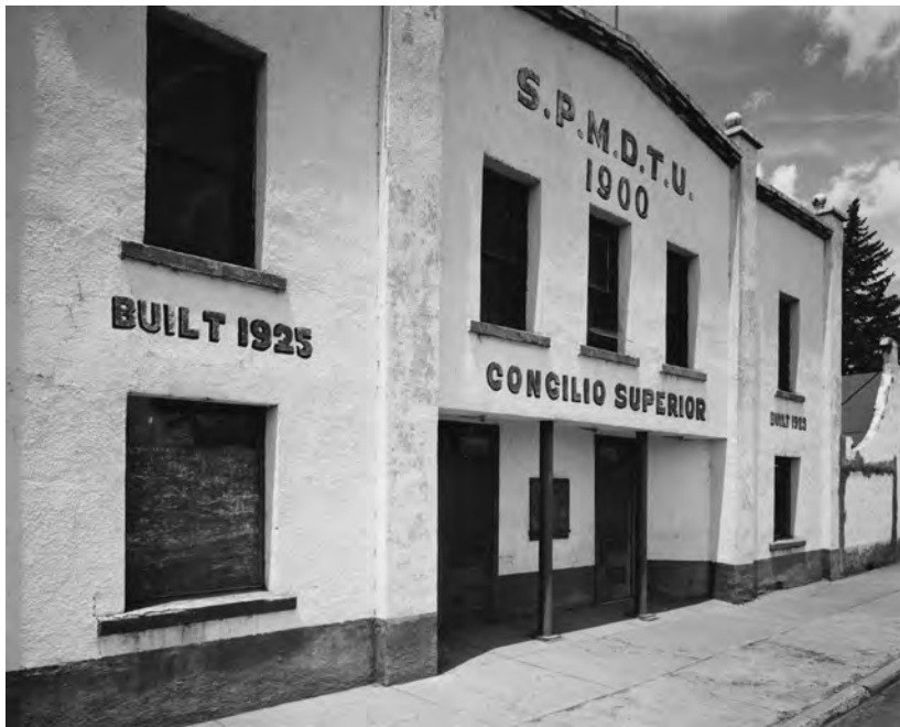
SPMDTU Building, Antonito, Colorado. Denver Public Library Auraria Collection. Photographer: Daniel Salazar, Denver, Colorado.
