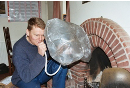
Figure 10. Use of a chimney balloon is a simple way to reduce air infiltration from a fireplace.
