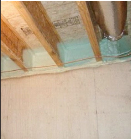
Figure 2. Spray foam seals leaks between floor joists and the foundation.
