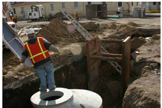
Development will require installation of new sewer lines.
