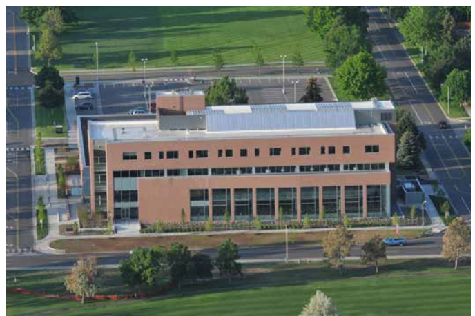
The Parade Grounds will connect to the Art Walk to the east as well as the Health and Wellness Center (shown above) to the north.
