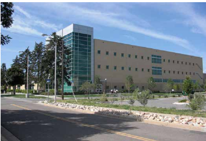
Campus Services Building.
