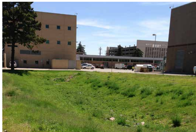
Retention pond north of CUP as seen from 19th Place and Victor Street.
