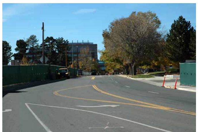
Seventeenth Place between Wheeling Street and Fitzsimons Parkway will need to be widened to accommodate five lanes of traffic.
