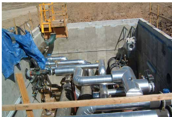
Installation of steam, condensate return, and chilled water lines in vault 11.
