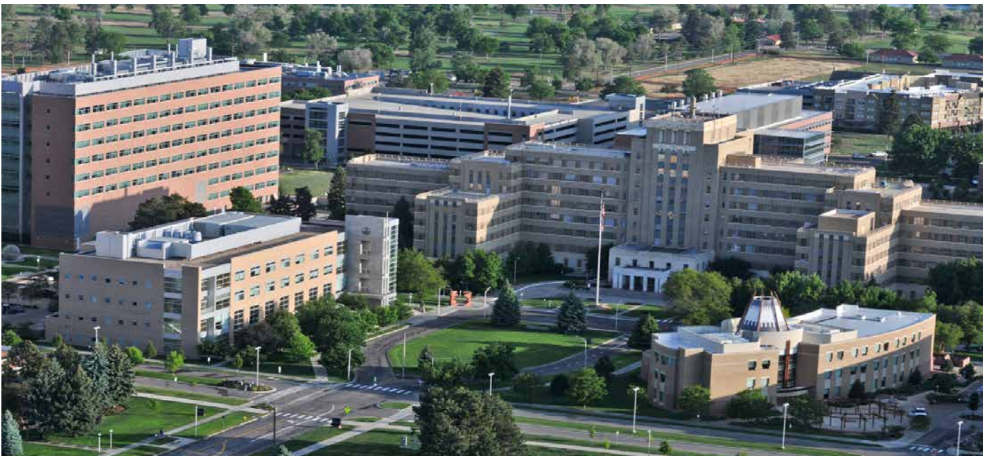
Bonfils Circle, the turnaround in front of Building 500 will become a ceremonial green space.
