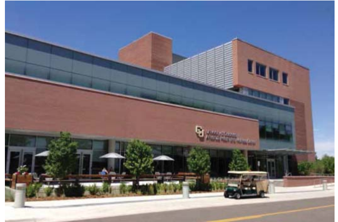
The Health and Wellness Center presents a clearly articulated entry condition along an activated streetscape.
