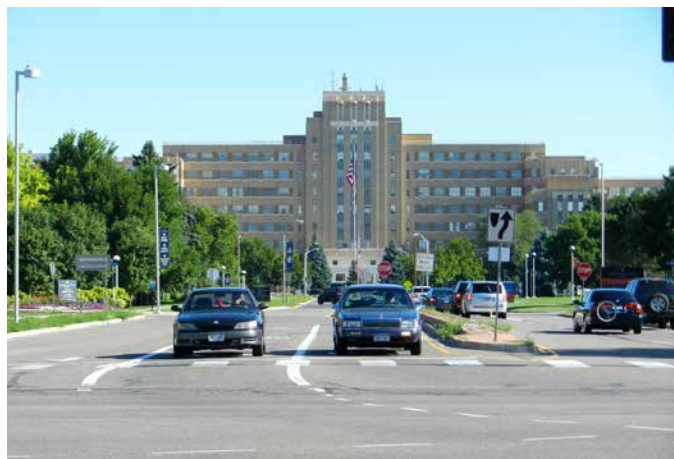
Aurora Court is an important point of access to the campus, both symbolically and in terms of traffic volumes.
