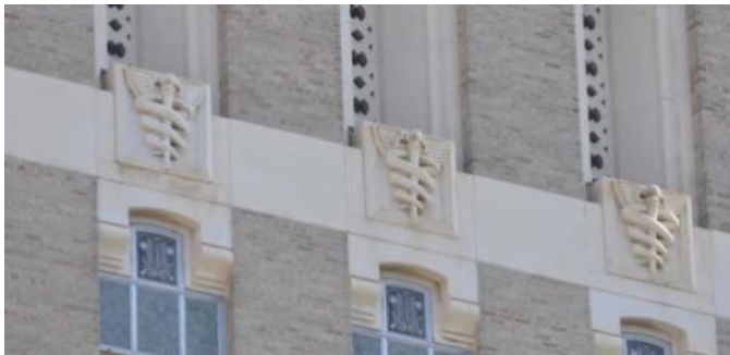
Building 500 exhibits a richness in architectural detail
