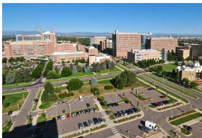
Much of the campus's parking need is met with surface parking.
