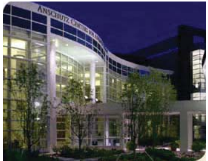
The curtainwall articulations on the UCH Anschutz Center for Advanced Medicine respond well to a human scale.
