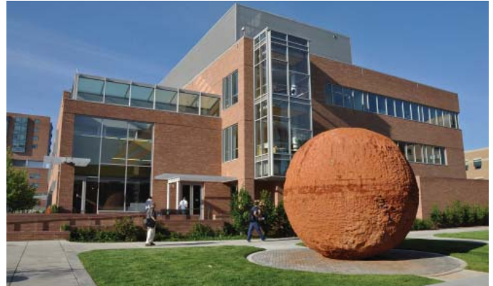
The School of Dental Medicine Building relates well in terms of scale and materiality with the adjacent Art Walk.
