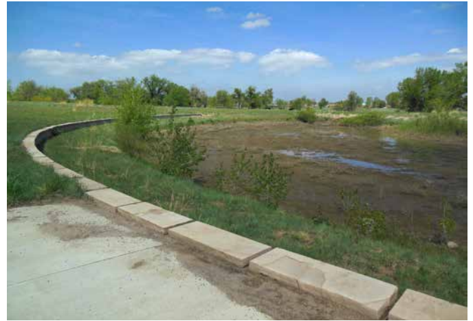
Detention ponds in Sand Creek hold excess capacity for special flood events.
