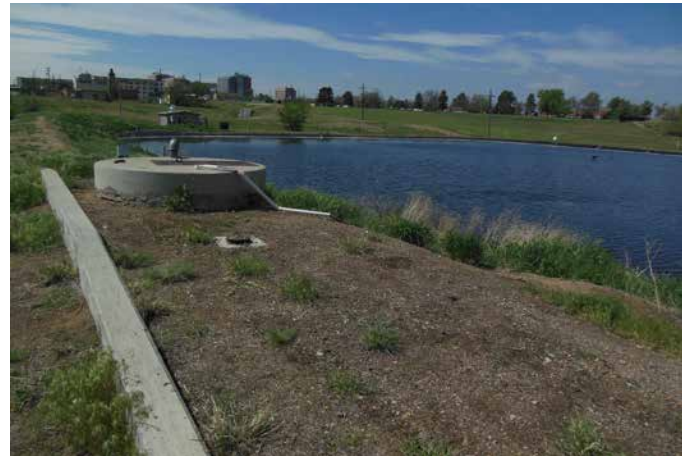
Regional Detention Pond 374.
