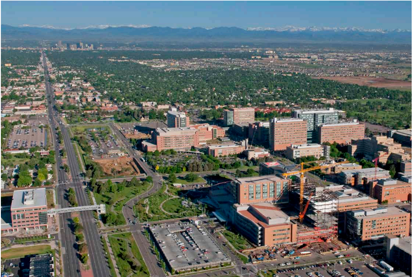
An exercise trail will develop in the landscape buffer on the northern edge of Colfax Avenue (roadway along left edge of photo).
