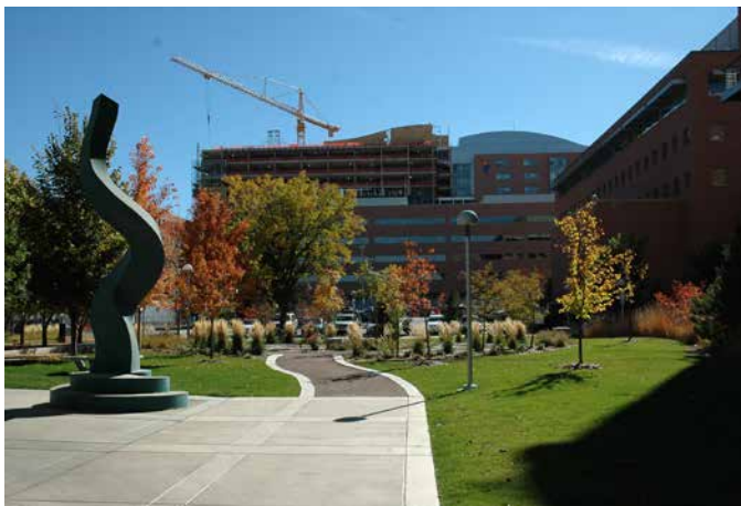
The garden between PASCAL and Education 2 North encapsulates desired qualities of flexibility and comfort, and frames views of CHCO, which contributes to wayfinding on the site.
