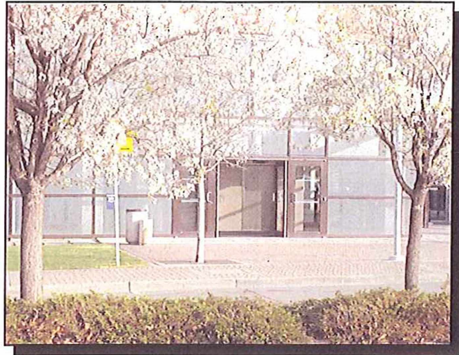
Once on the western edge, Auraria's only parking structure is now in the center of campus.
