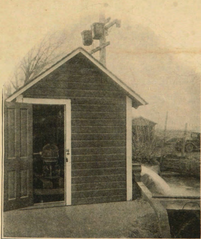
A VERTICAL TURBINE PUMP DIRECT CONNECTED TO AN ELECTRIC MOTOR.
