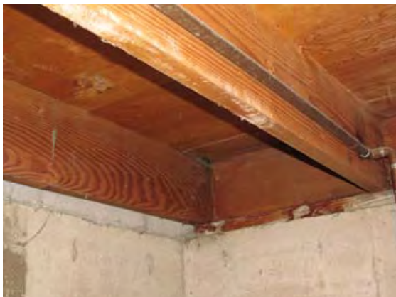
A typical uninsulated basement in a 40-year-old home.
