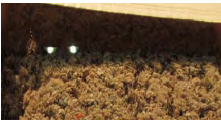
Blown Cellulose: R3.2-R3.8 per inch Cost: $.70 to $2.00 per sq. ft. installed
