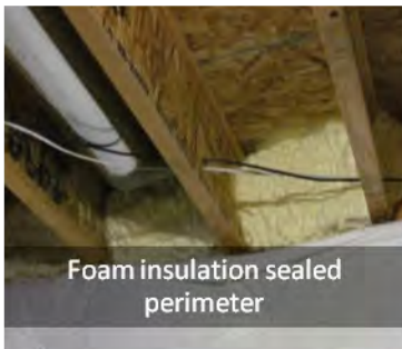
Conditioned attic (ceiling has spray foam)
