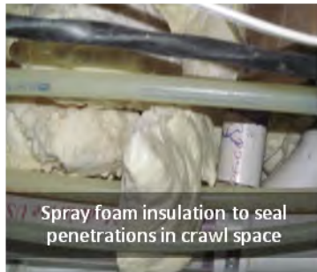
Sprayed foamed rim joists and penetrations in crawlspace
