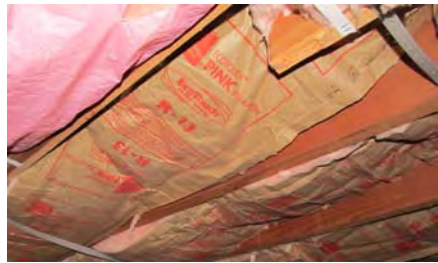
Fiberglass Batt: R3.2-R3.8 per inch Cost: $.70-$2.00 per sq. ft. installed
