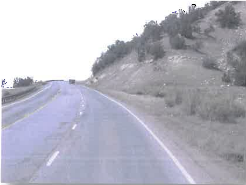
Milepost 4.4, Right turn lane and passing lane approaching Bondad Hill
