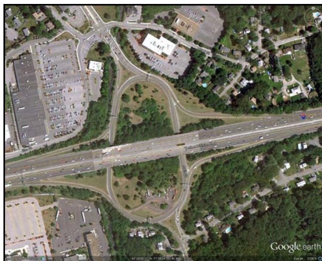
Figure 2-19. Aerial Photo of a Two-Level Roundabout Interchange with a Circular Roundabout in Massachusetts
