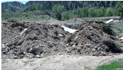
Picture 1. Topsoil Stockpile for the I-70 Eagle project.
