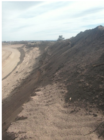
Picture 5. No wind or water erosion on topsoil piles.
