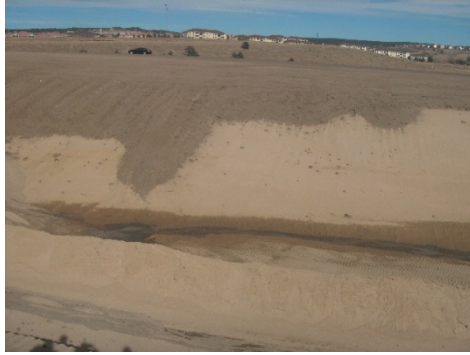
Picture 6. Topsoil spreading in progress.
