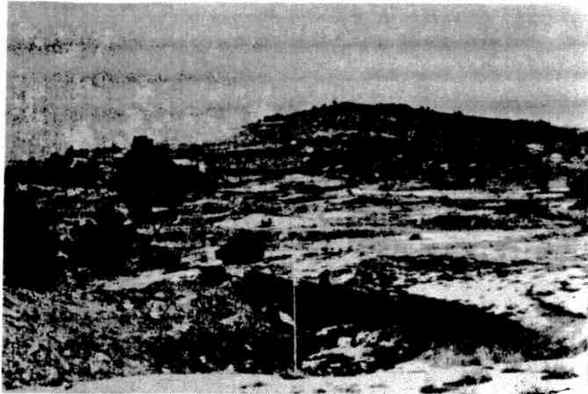
Figure 7. Collapse over room of Marshall No. 1 mine. The collapse area is approximately 15 feet by 30 feet and is about three feet deep. From five to ten feet of coal were extracted from this area at a depth of about 50 feet. Lower slopes of hill in background are also shown in Figures 6 (Area A), 8, 31, and 32. Locality 4, subsidence-inventory map.
