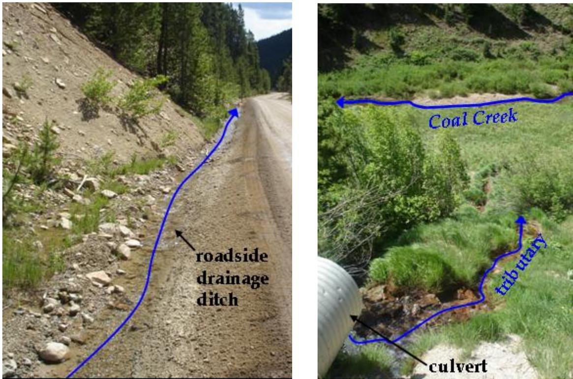
**Figure 6.** Water seeping from a hillside along County Road 12 on the north bank of Coal Creek (which is located to the right of the road) is diverted to a ditch which carries the water to a culvert crossing under the road further downstream (left). Water exiting a culvert under County Road 12 is dispersed into a marshy area on the north bank of Coal Creek (right). In these cases, samples were taken directly from the culvert.
