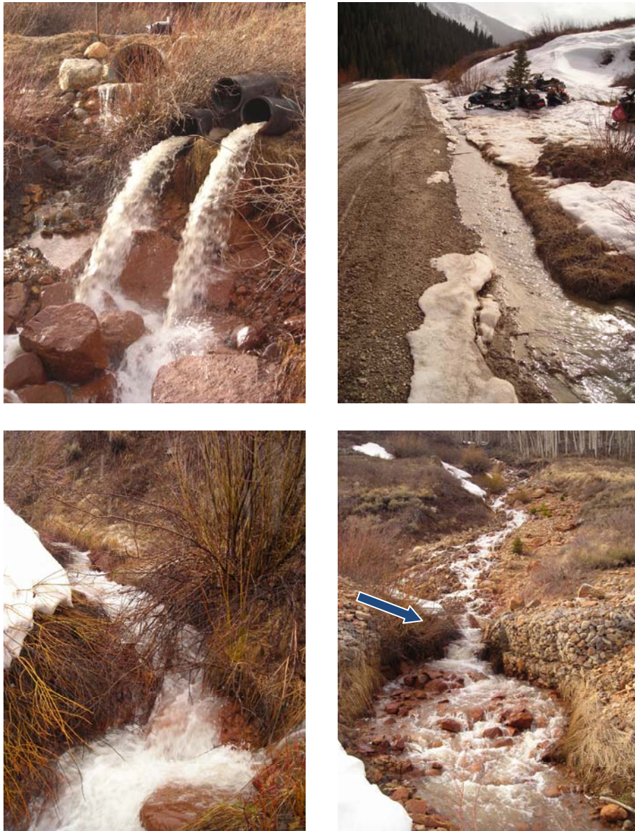
Figure 30. Photographs of the drainages combining to make up the tributary UT-5.368: (upper left) view from the south side of County Road 12 where the oval culvert in left background drains the road-side ditch and the cast-iron pipes drain the treatment plant effluent and the Keystone Mine drainage; (upper right) view of the road-side ditch on the north side of County Road 12 which drains through the oval culvert; (lower left) close-up view of the Mount Emmons treatment plant effluent; and (lower right) the Keystone Mine drainage which is joined by the treatment plant effluent at the blue arrow.
