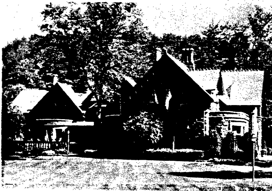
Figure 1. Briarhurst Inn constructed in 1874 by Dr. William Bell is located between El Paso Boulevard and Fountain Creek.
