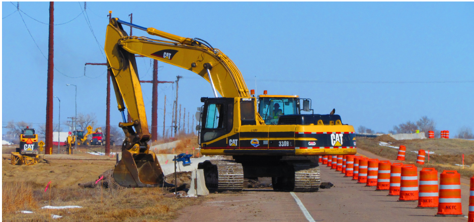
Highway construction cone zone on I-76
