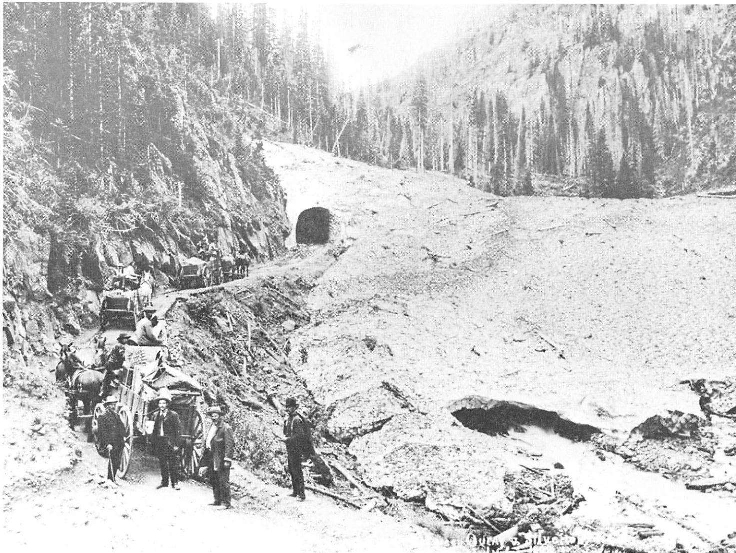
Frontispiece. July 1888 photograph of a hand-dug tunnel through the winter debris deposited by the East Riverside avalanche. Numerous mature coniferous trees brought down by the avalanche are scattered throughout the deposit and Red Mountain Creek flows through the debris. (San Juan County Historical Society)
