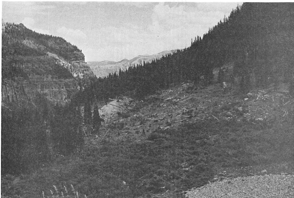
Figure 5. Earthen dam located just back from the cliff edge above the Camp Bird Mill. The dam was constructed shortly after the mill was destroyed by an avalanche on 17 March 1906. This photograph, taken in July 1976, shows large trees deposited against the uphill side of the dam by an avalanche from U.S. Basin on 9 January 1974. (B. Armstrong photo)
