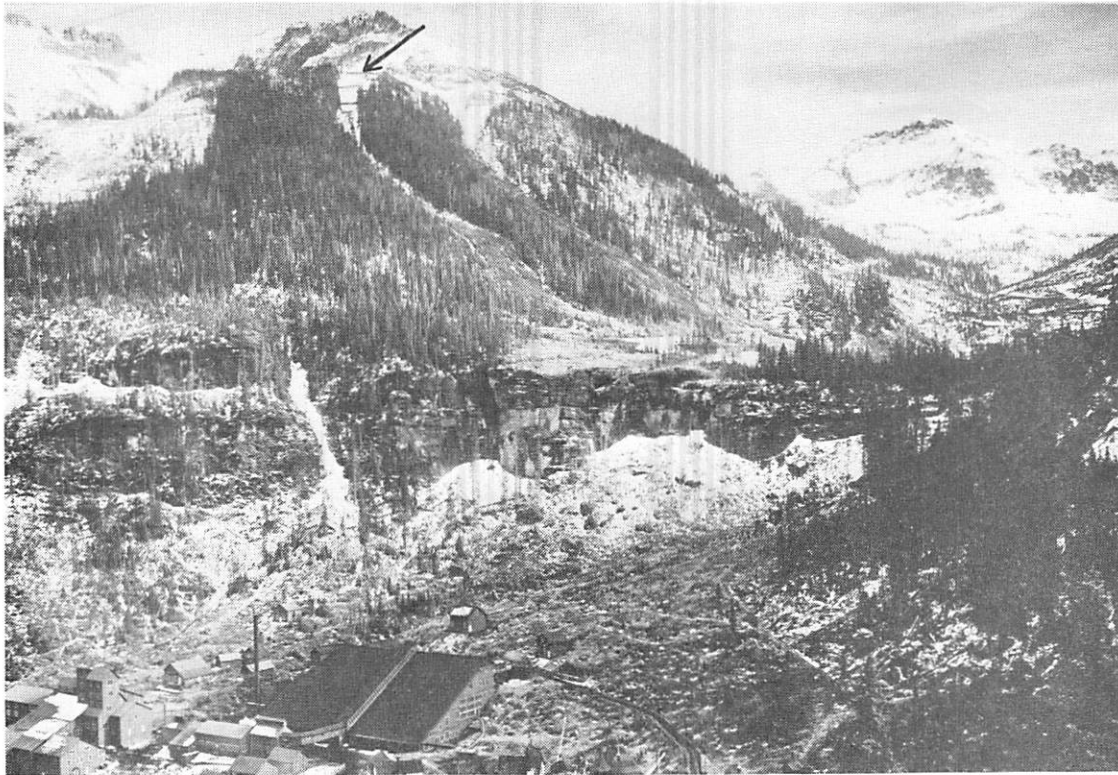
Figure 26. The rebuilt Camp Bird Mill, circa 1912, showing the lower path of the U.S. avalanche, entering on the right, and the two Mt. Hayden avalanche paths. On 17 March 1906, the U.S. avalanche and possibly one of the Mt. Hayden paths released to destroy the mill and the tramway, leaving only a few standing trees directly underneath the cliff band. Note the supporting structures in the starting zone of the left Mt. Hayden path. (Denver Pub. Lib., West. Hist. Dept.)
