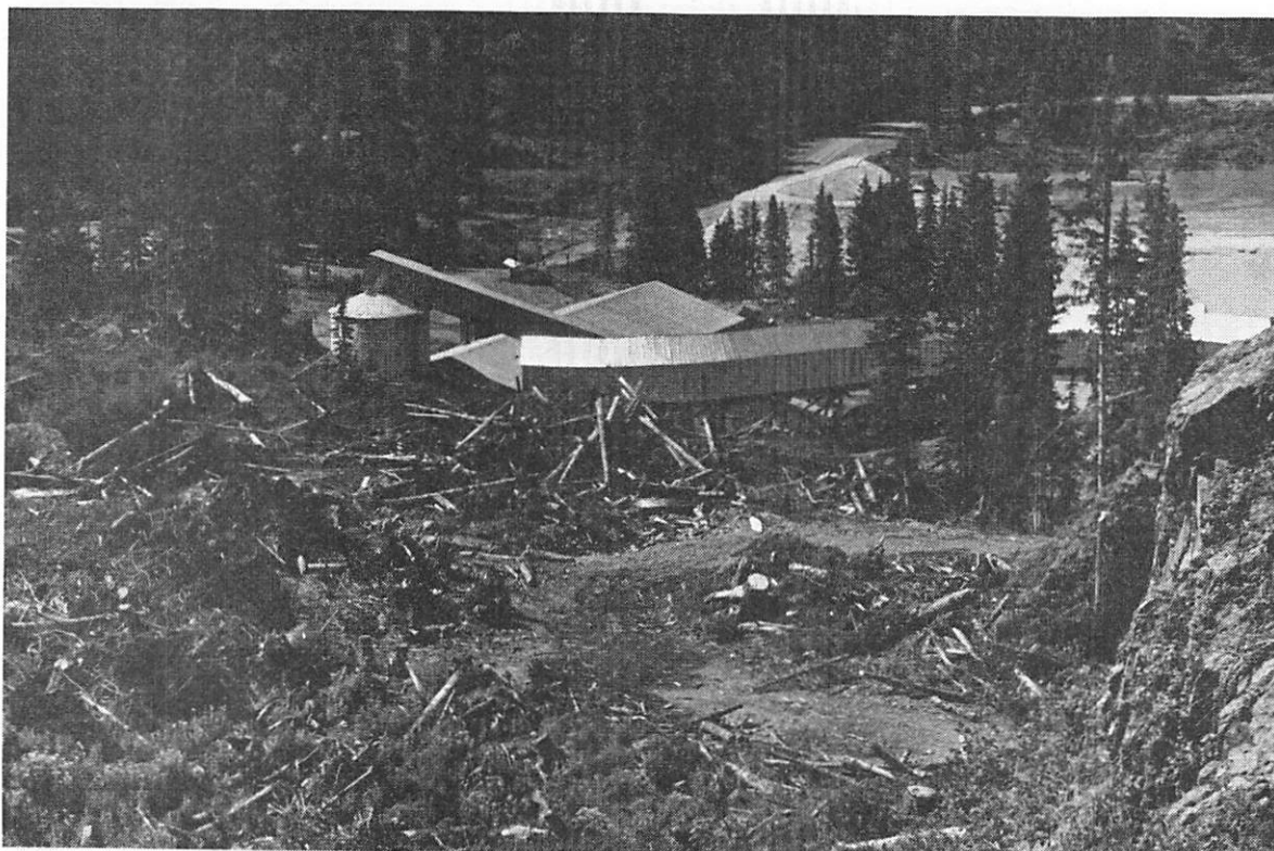
Figure 30. The Camp Bird Mill, July 1976, viewed from just downslope of the cliff band. Uprooted timber deposited by the 1974 avalanche still remains. (B. Armstrong photo)
