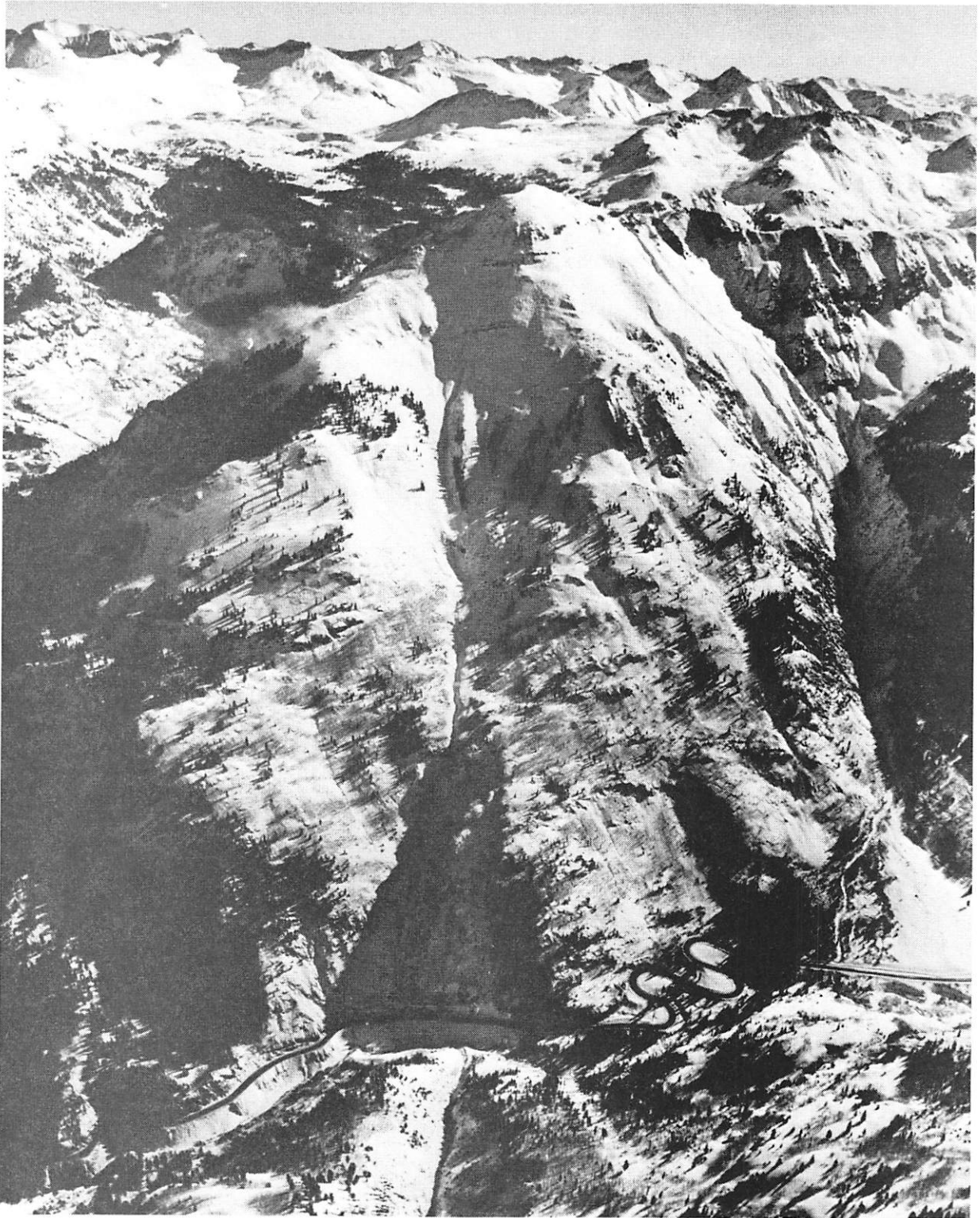
Figure 32. East Riverside avalanche path, U.S. Highway 550. (INSTAAR photo)
