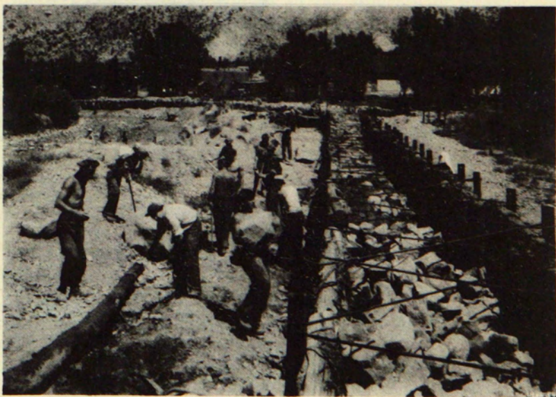
CCC BOYS WORK ON REVETMENT TO PROTECT CITY PROPERTY.
