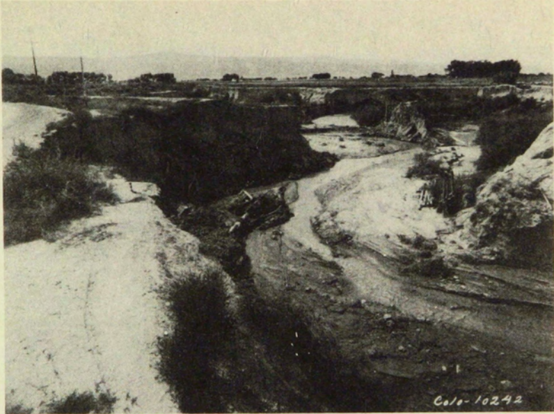
B. BRIXNER LOSS OF VALUABLE FARM LAND. ROAD ENDANGERED. RESULTS IN INCREASED TAXES FOR MAINTENANCE.
