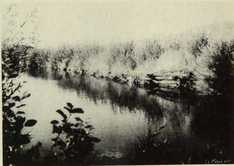
BANK STRUCTURE (REVTMENT) AND WILLOW PLANTING, PREVENT CUTTING OF ADJOINING LAND.
