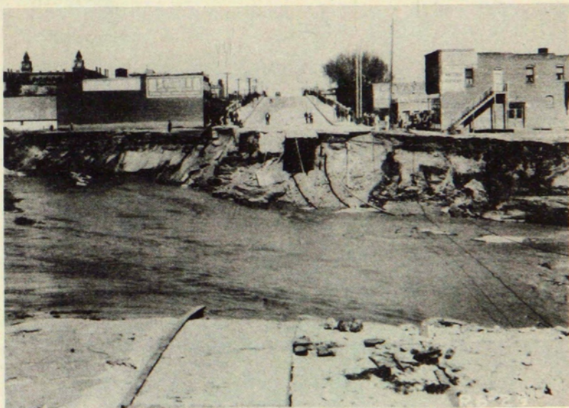
FLOOD DAMAGE, IN COLORADO, 1935.
