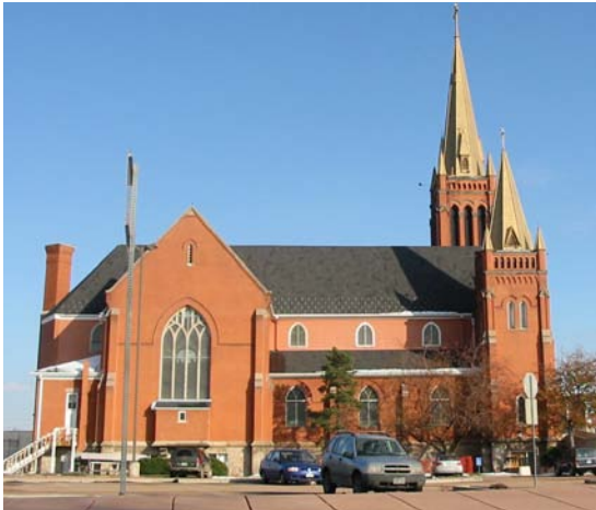
Figure 2-66. St. Mary's Cathedral, one of the region's culturally important buildings, stands astride Bijou Street, a key gateway entrance into downtown Colorado Springs.
