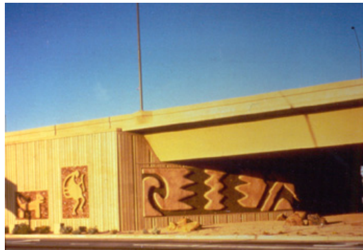
Sample of Phoenix art work at bridge retaining wall.
