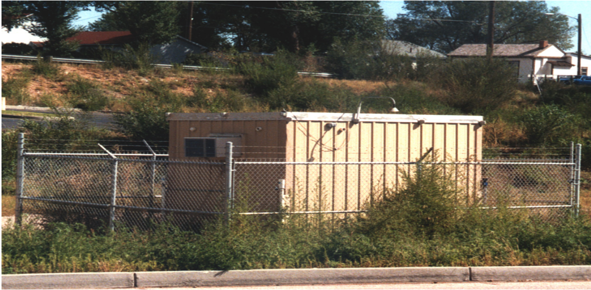
Figure 2-53. Monitoring stations in key areas of the region help keep track of air pollution concentrations.
