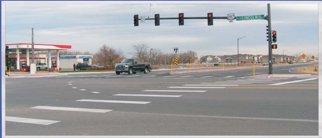
View east along SH 402 at US 287
