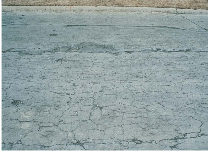
Figure 52 - Map Cracking
