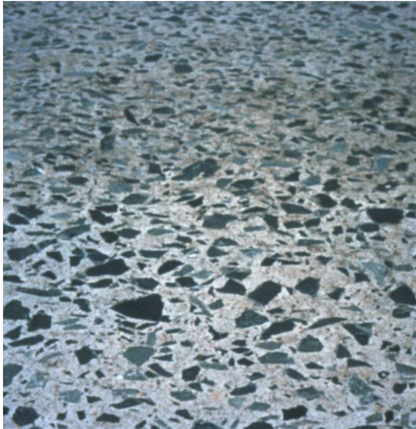
Figure 55 - Polished Aggregate
