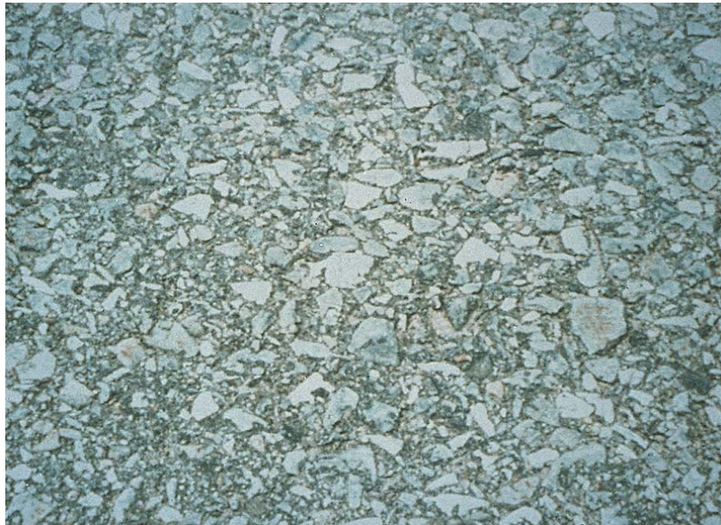
Figure 28 - Polished Aggregate
