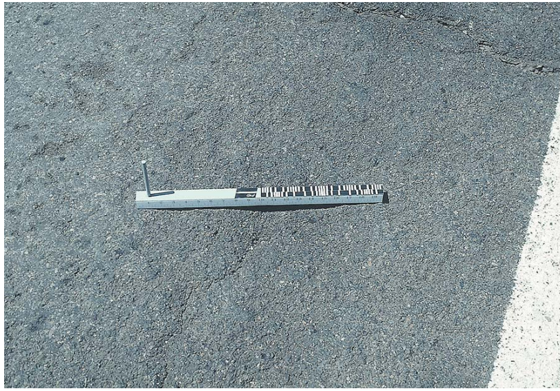
Figure29 - Loss of Fine Aggregate
