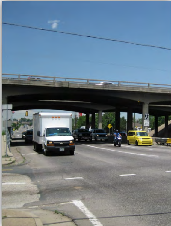
Kipling Street under I-70 bridges
