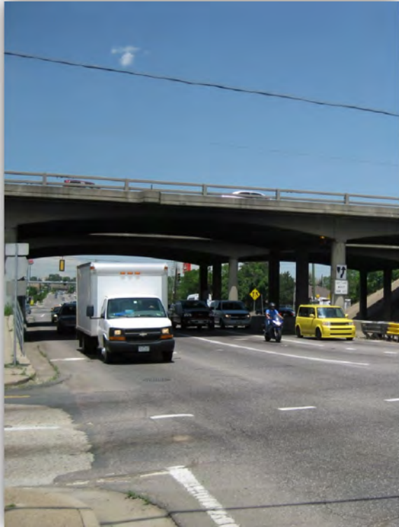
Kipling Street under I-70 bridges
