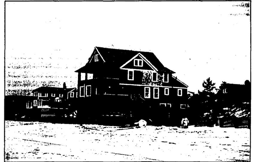
Figure 7.1 (c). By 1987, the dune line has receded behind the house, leaving it entirely on the beach. House was washed away on October 31, 1991. (Photo by R. Platt.)
