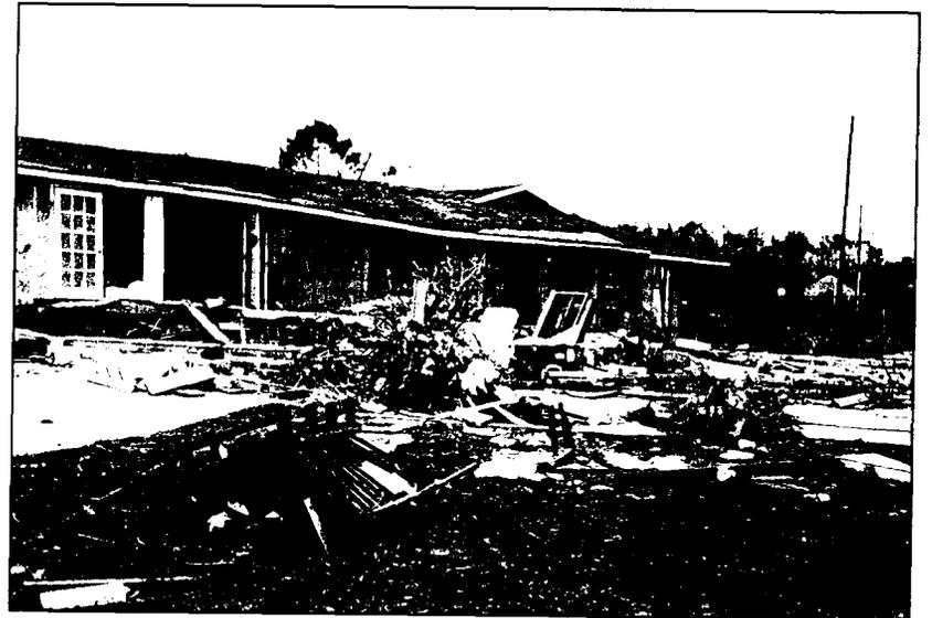
Figure 5.5. This house on the Isle of Palms was moved landward off its foundation by Hurricane Hugo. (Photo by R. Platt.)
