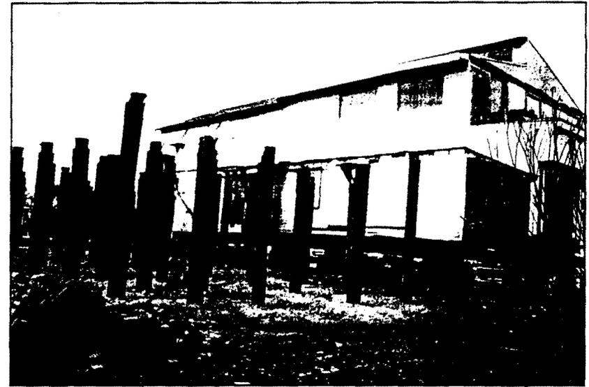
Figure 5.8. House-movers lifted many houses upward and sideways, but not usually landward from eroding shorelines. (Photo by R. Platt.)
