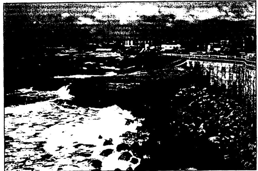
Figure 1.5. Riprap installed in San Diego to mitigate wave damage to shore road after natural rock shoreline has eroded away. (Photo by R. Platt)
