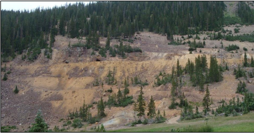
Photo 23. The Daisy Mine in Redwell Basin. The collapsed adit is in the foreground of the photo. An access road to the Peeler Lake Trail passes through several waste rock piles. Gunsight Pass Road is near the top of the photo. Photo courtesy of Ashley Bembenek.
