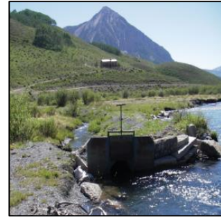
Photo 20. An irrigation head gate in the Slate River.
