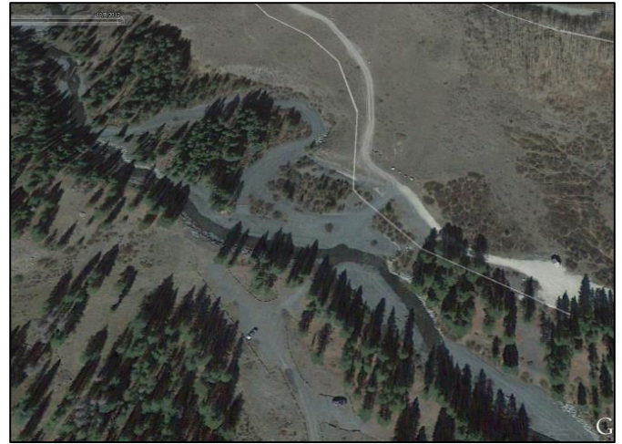
Photo 8. The Slate River near Oh-Be-Joyful Campground in 2012. Note the new channel alignment through the forest; flows no longer pass through the meander bend, and large boulders armor the banks along the new channel in the forest and the Campground. Image courtesy of Google Earth and the USDA Farm Service Agency (2012).
