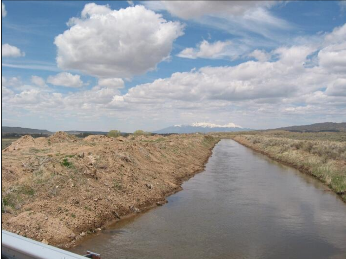
Figure 4-7. Upstream view of Sanchez Canal at the J8 Road Crossing, Showing Dredge Spoil Placed along the Berm
