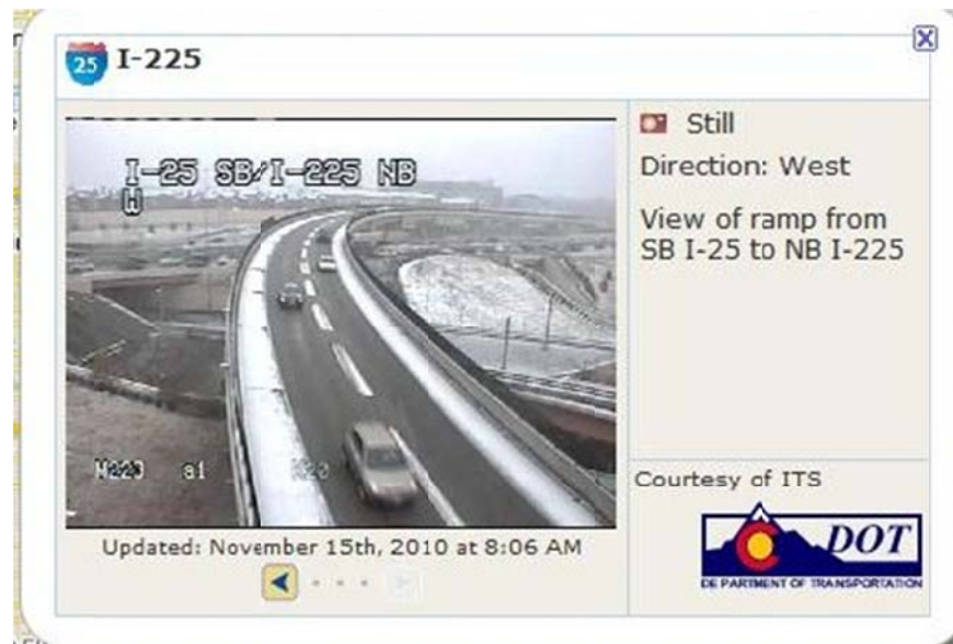
Figure 7.7.3: I-25 / I-225 Spray System Activation (CDOT, 2010)
