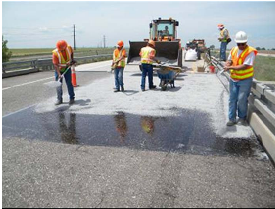
Figure 6.1.2.2: SafeLane Aggregate Being Placed by Hand
