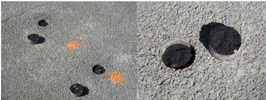
Figure 7.4.1.2: Asphalt Bond Test Failure Modes
