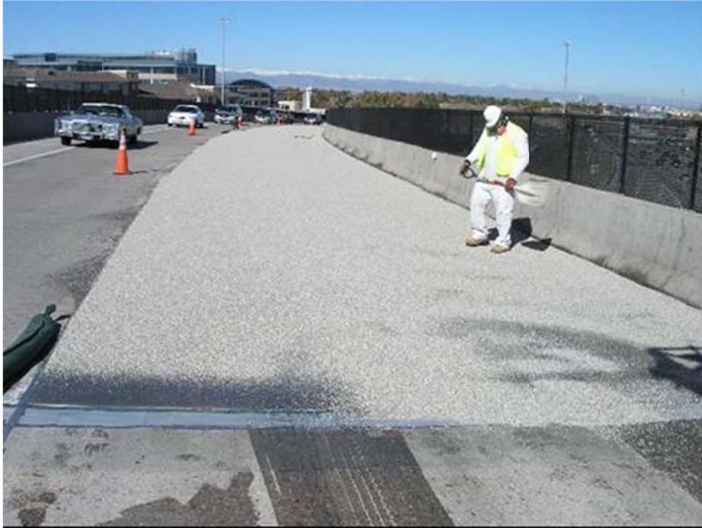
Figure 6.2.3.3: Flexogrid Aggregate Being Spread by Hand
