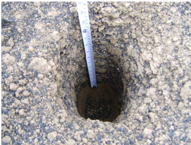
Figure 11. Inspection borehole in a 300-mm-thick ESR layer compacted with regular field equipment (Rubber content: 20%, Target relative compaction: 95% of maximum dry unit weight obtained with standard compaction effort)
