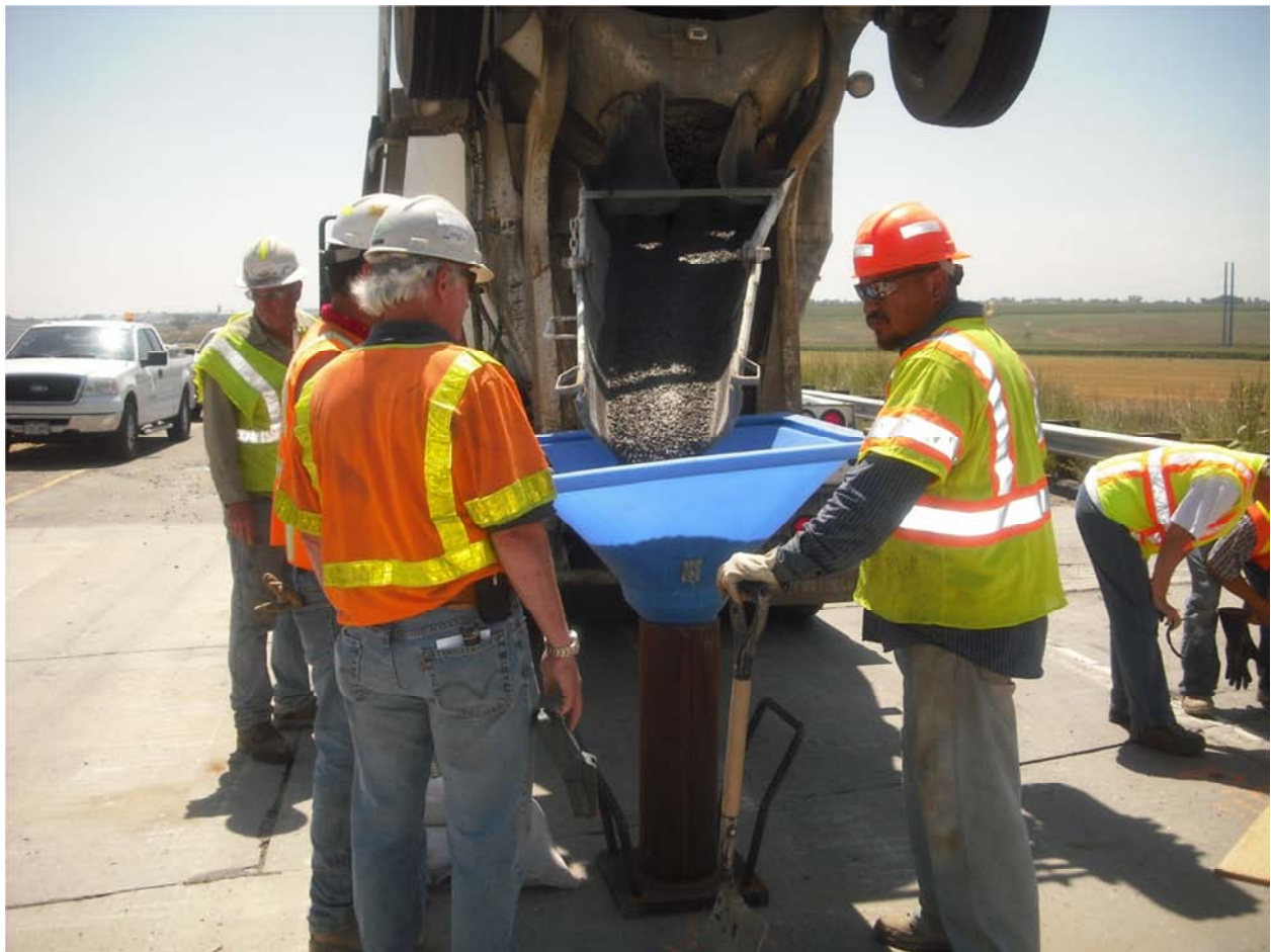
Figure 2: SCC Placement Funnel
