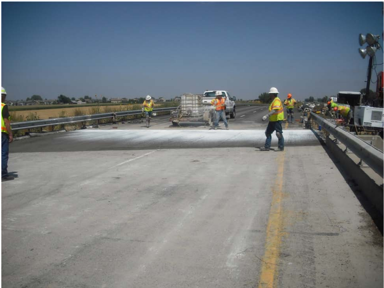
Figure 1: Southbound Bridge, North Abutment
