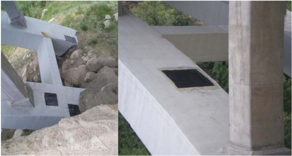
Figure 3.27. The repaired sections on the north end of the arches
