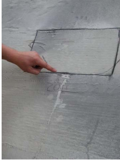
Figure 3.21. Water exiting the void area directly after the lower cut through the CFRP was completed
