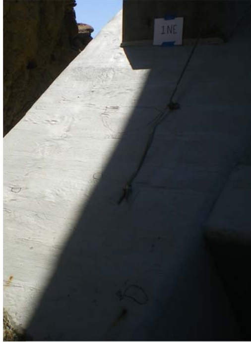
Figure A3. Bay 1NE, 5 voids
