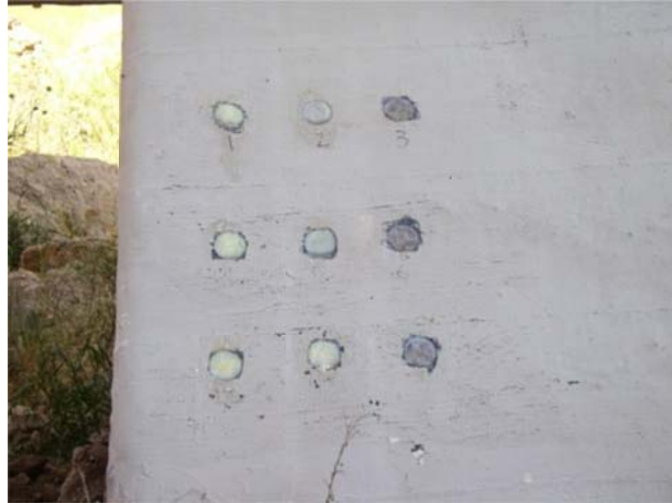
Figure 3.24. Epoxy filled holes following the pull-off tests
