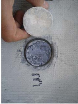
Figure B3. Test No.3, Photograph of test No.4 is not available
