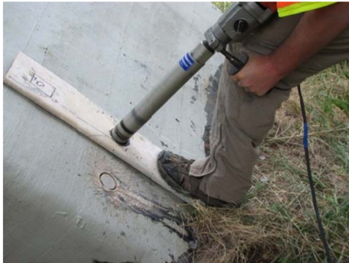
Figure 3.5. Starting a core hole using a wooden jig
