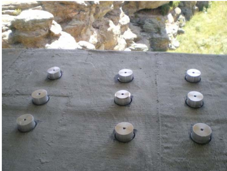
Figure 3.11. Adhered aluminum pucks for pull-off tests
