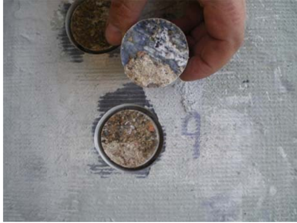
Figure B8. Test No.9, weak bond strength
