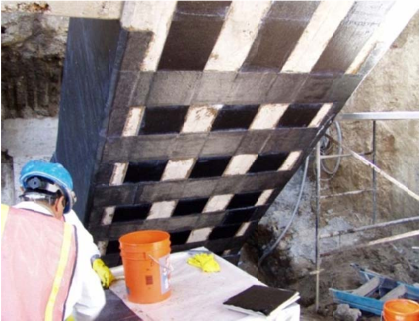
Figure 2.11. Longitudinal and transverse CFRP wraps at the base of an arch (Mohseni, CDOT)
