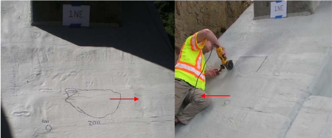
Figure 3.20. Void in CFRP with transverse crack identified with red arrows and cutting the perimeter of the void in the CFRP
