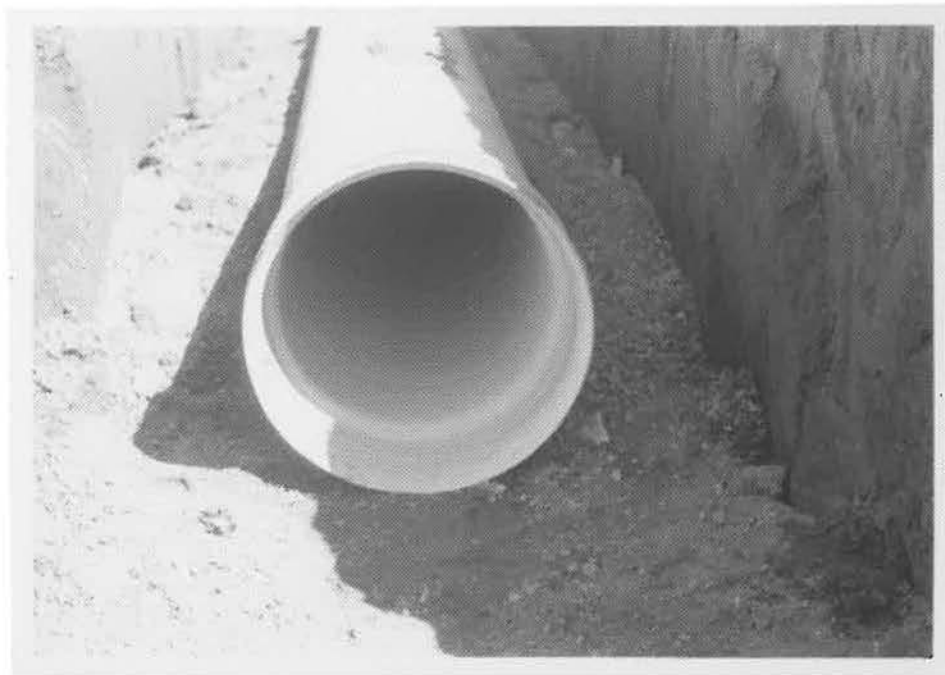
Photo 4. 21" Pipe at grade in bottom of trench.
