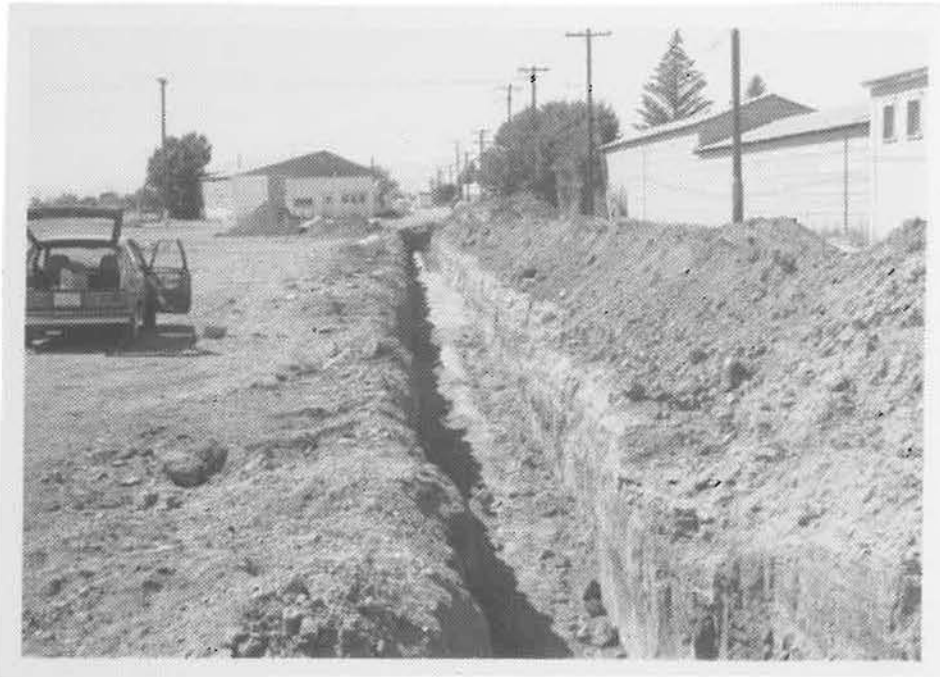
Photo 6. 21" Pipe after backfill.
