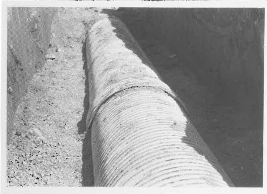
Photo 5. 21" JM PVC Sewer Pipe. Backfill partially completed.
