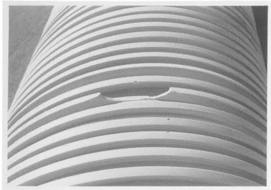
Photo 3. 21" JM PVC Sewer Pipe. Pipe was easily chipped if mishandled.
