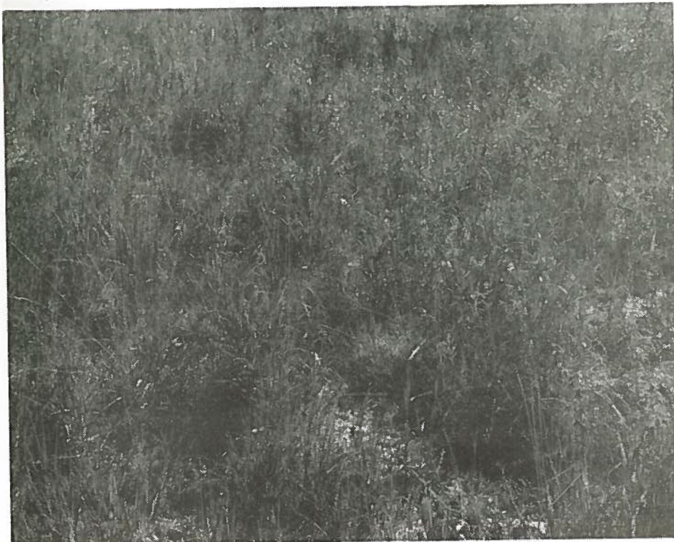
Photo No. 8. Taken 7/24/78 Vail Pass Hold-Gro, Sta. 645+50 Installation Date: 10/15/76 Hold-Gro on left, standard jute on right, junction just left of center of photo.
