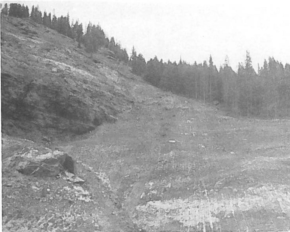
Photo No. 2 Taken 6/27/78 Same site as Photo No. 1 Shows rock and mud slide from above partially covering test site
