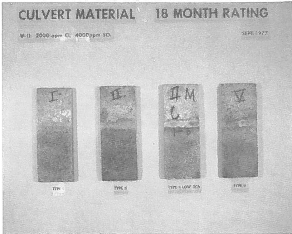
Photograph No. 17 Concrete samples after 18 months in a harsh water environment
