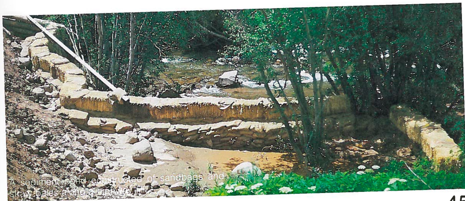
Sediment was very visible in the streams where erosion control features failed.
