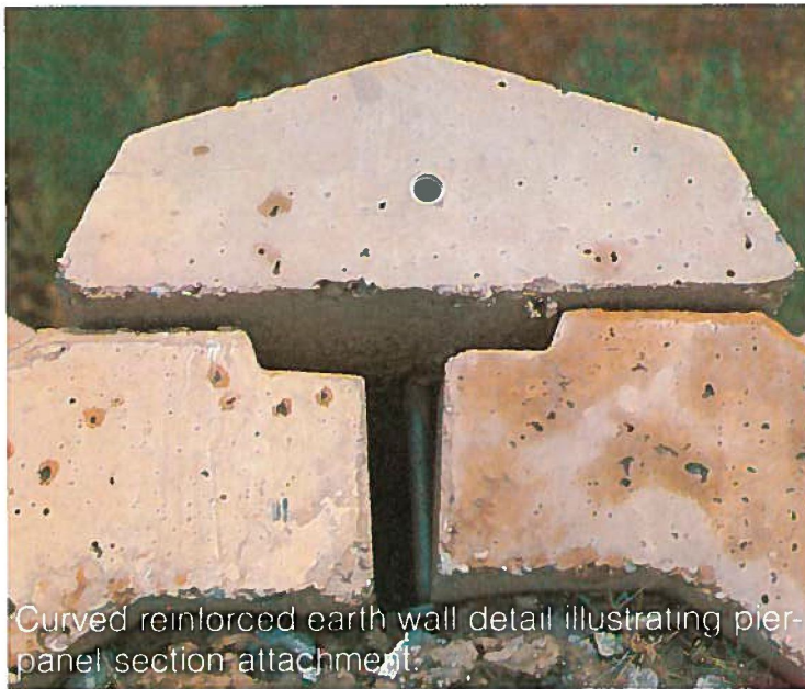
Details of retaining wall construction. Curved panel sections slip between the tieback sections.
