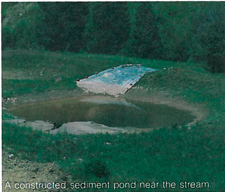
Old highway ditches were sometimes used as sediment ponds. Stand pipes were attached to existing culverts to increase the ponds capacity.
