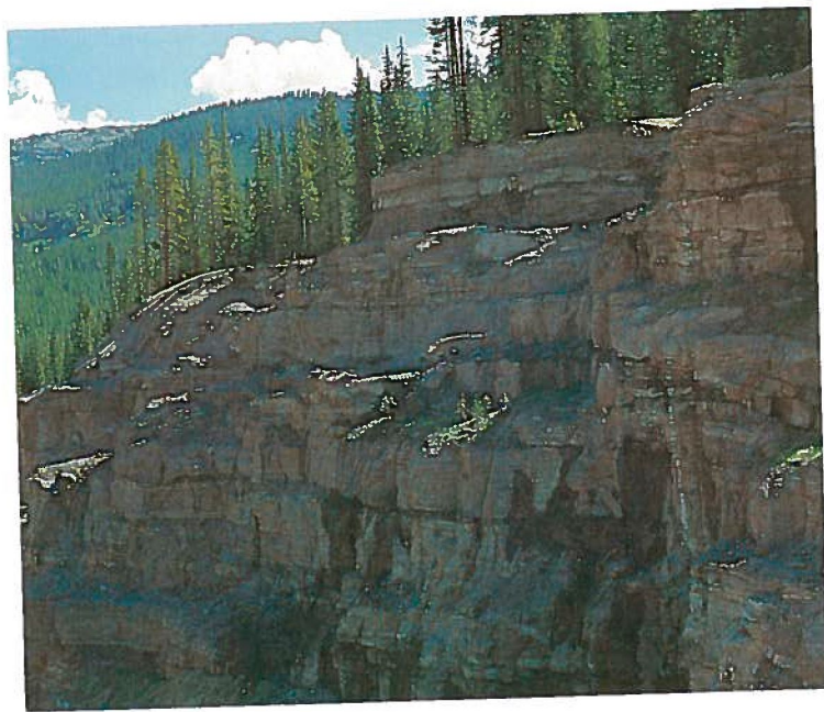
Natural appearance of rock cut immediately after blasting and cleanup.
