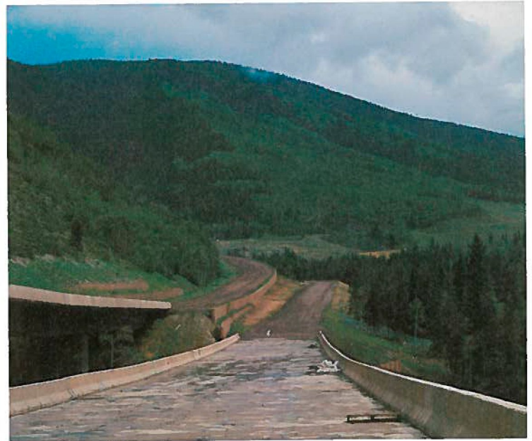
Land forms were blended with the bridge abutments to maintain visual continuity for the motorists.
