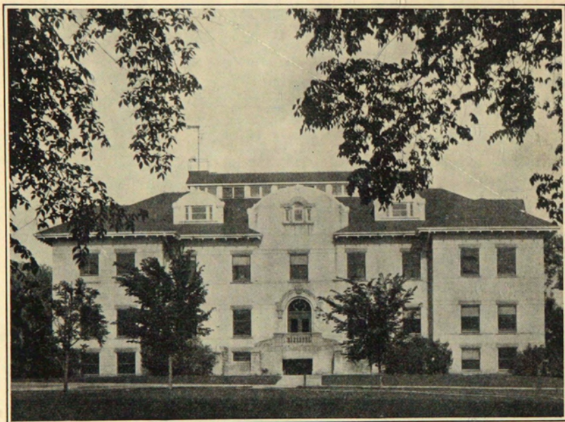
Fig. 2.—The Civil Engineering Building.
