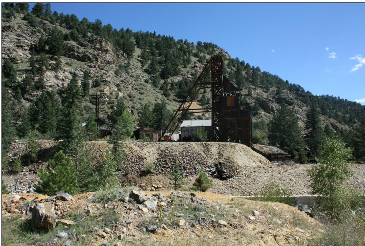
**Figure 59. View of Maude Munroe Mine Site (5CC.339) from Stanley Road with Headframe to the Right and Outbuildings to the Left. Log crib walls below headframe and concrete retaining wall at the creek are also visible; view to northeast.**
