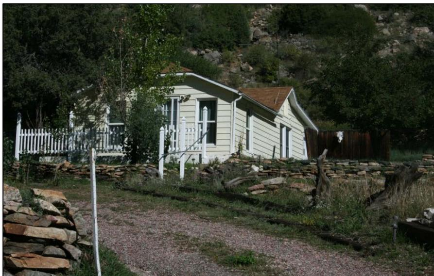
**Figure 50. View to North of South Primary and East Facades of 1615 County Road 308 (5CC.2153). Note the south primary facade shown in the photo is the 1938 addition, and the original block is visible under the roof gable of the east facade in the photo. The original block also is seen in the historic photos in Figure 51.**
